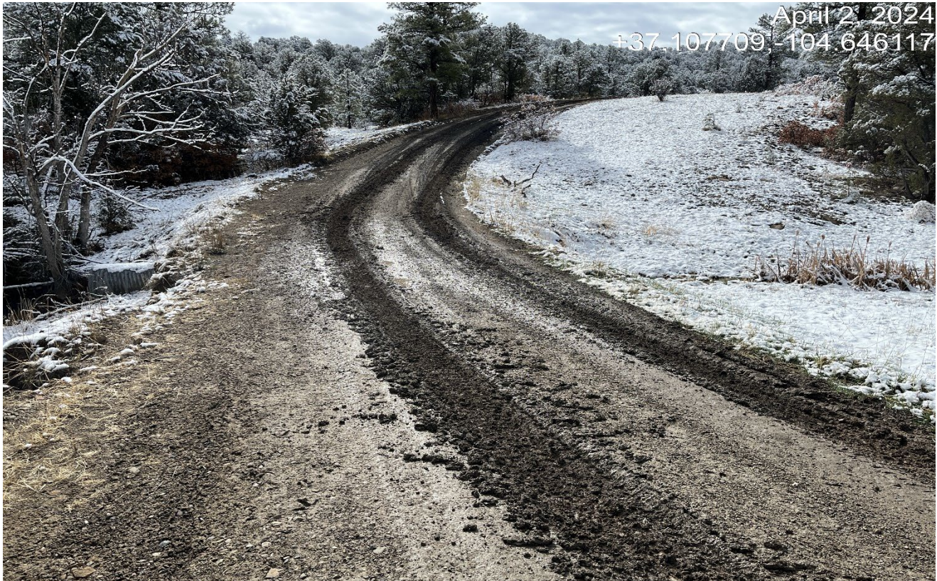
Photo 1. Facing southwest along the access road. There is vehicle rutting along the road which is slick and may need more gravel for stabilization.
