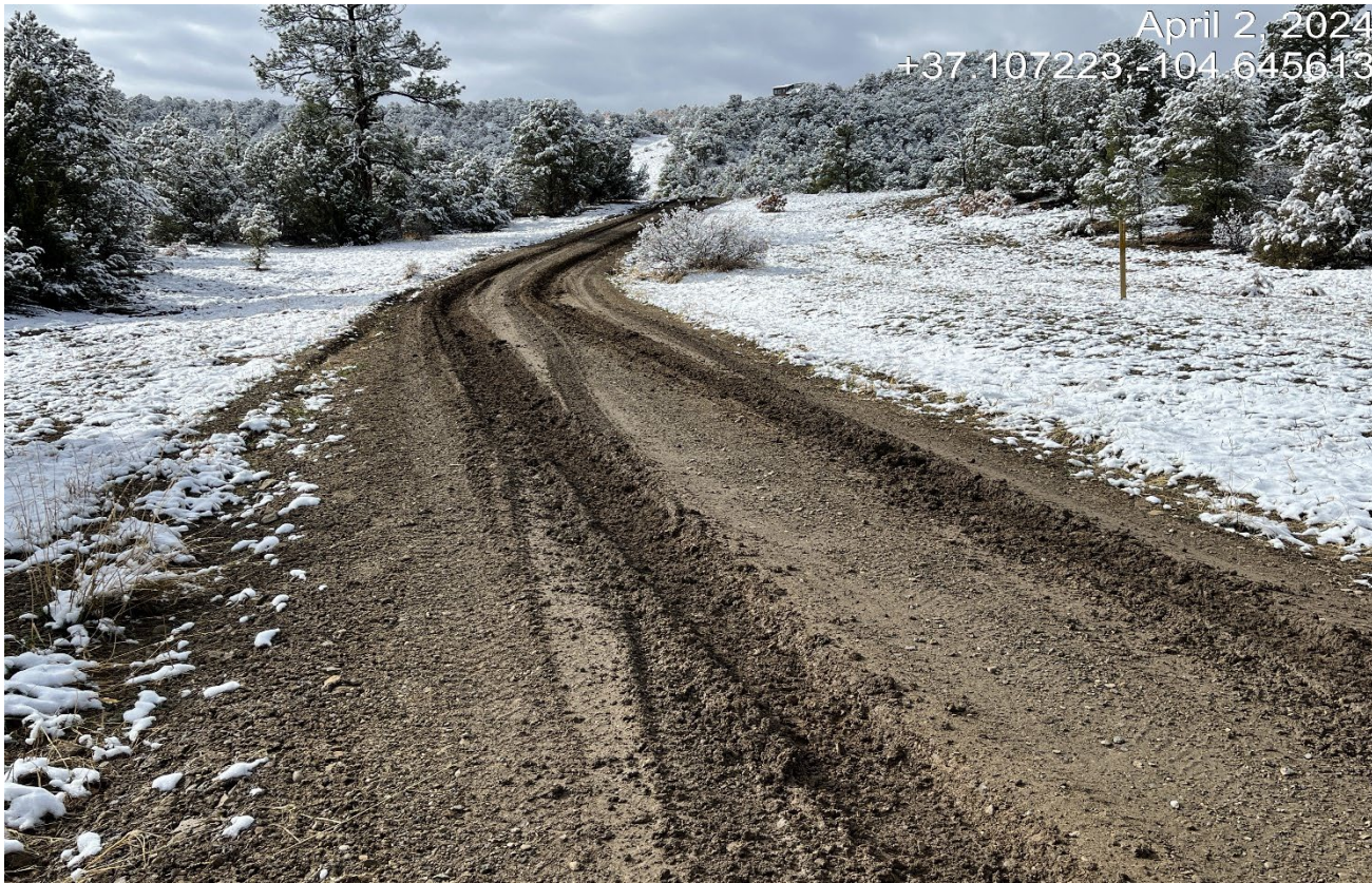
Photo 2. Facing southwest along the access road. There is vehicle rutting along the road which is slick and may need more gravel for stabilization.
