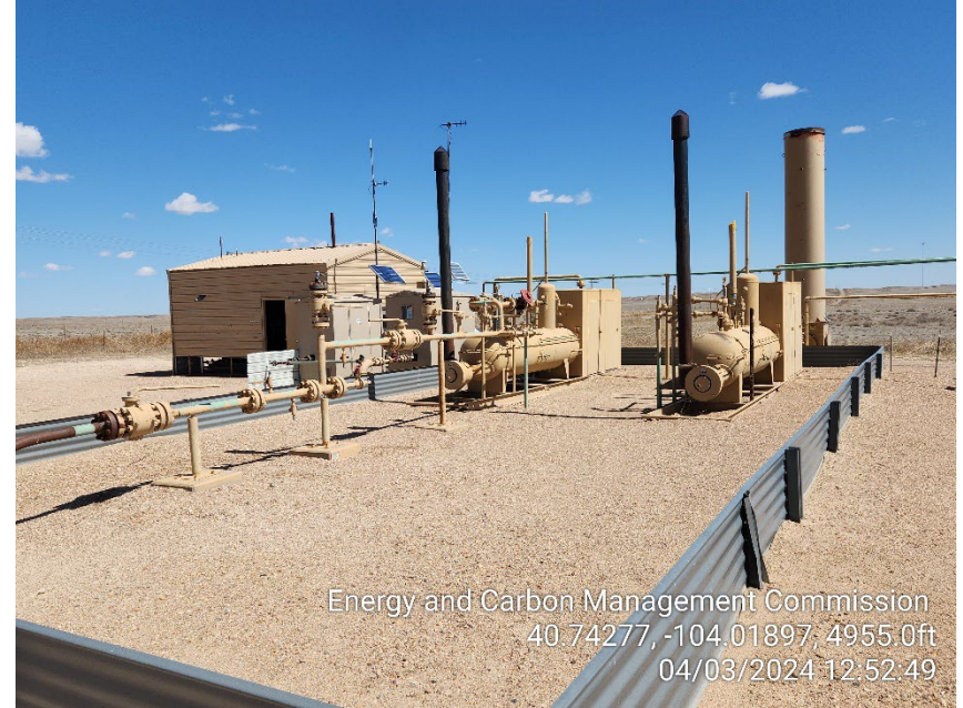
Photo 2 – Separators and ECD
