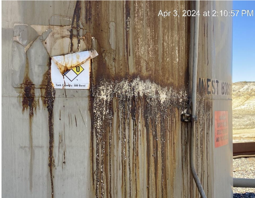
Illegible label. Tank overflow.
