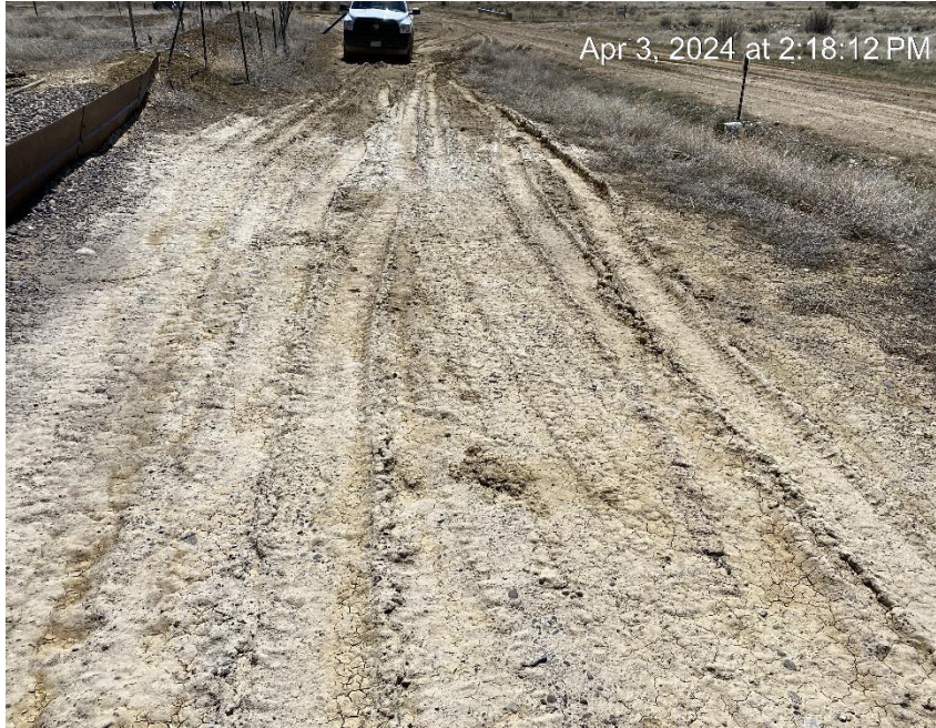
Sediment migration. Vehicle tracking.
