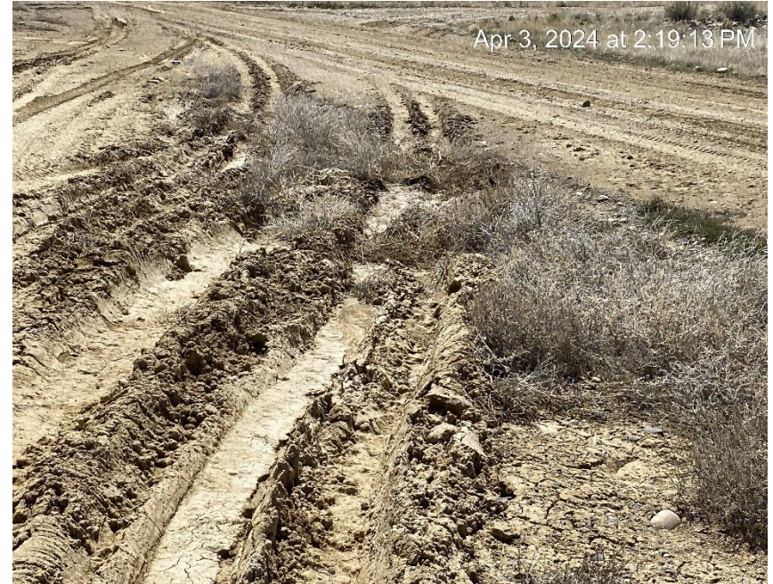
Sediment migration. Vehicle tracking.
