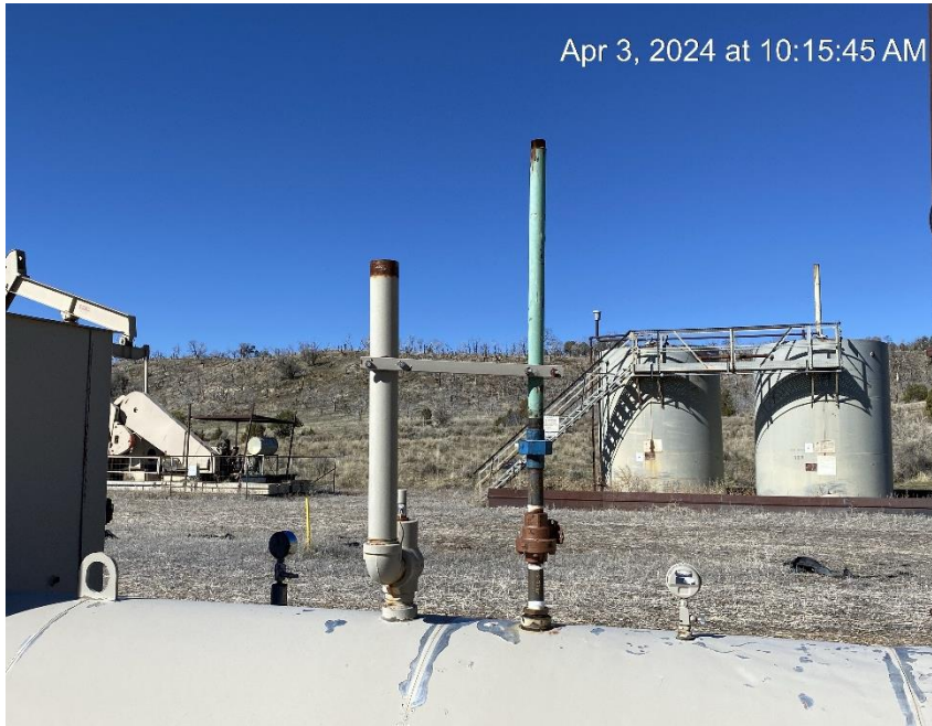
Relief risers missing rain protection
