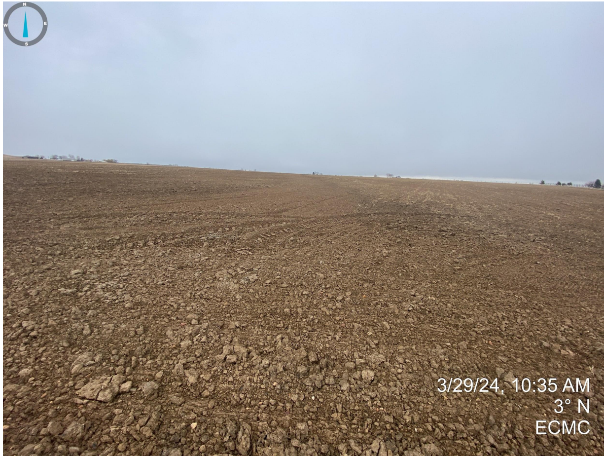
Photo 2. Taken from the southern portion of the former access road. Road base material has been removed and the former access road has been contoured/graded to match existing ag field.
