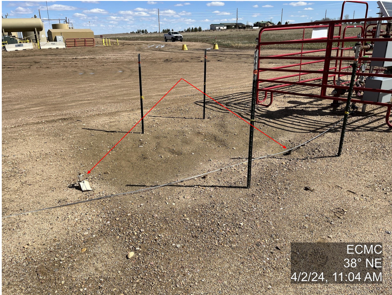
Photo 3. The photo was taken at the well location facing Northeast. The photo illustrates two risers that remain at the plugged and abandoned well location.
