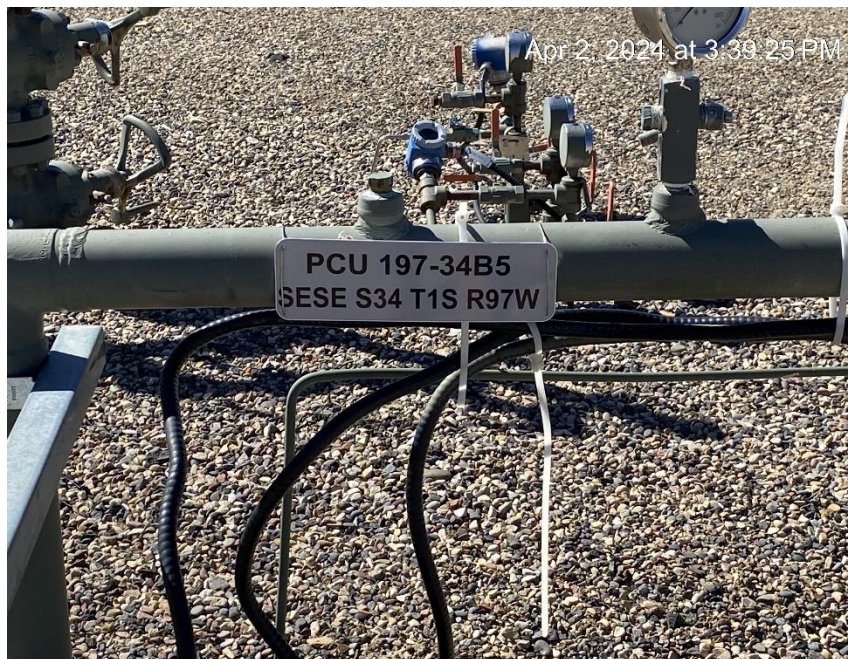
Wellhead sign missing required information
