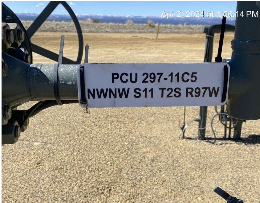
Wellhead signs missing required information
