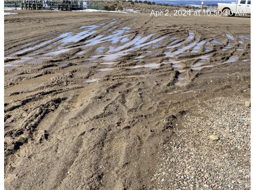
Lack of stabilization. Vehicle tracking.
