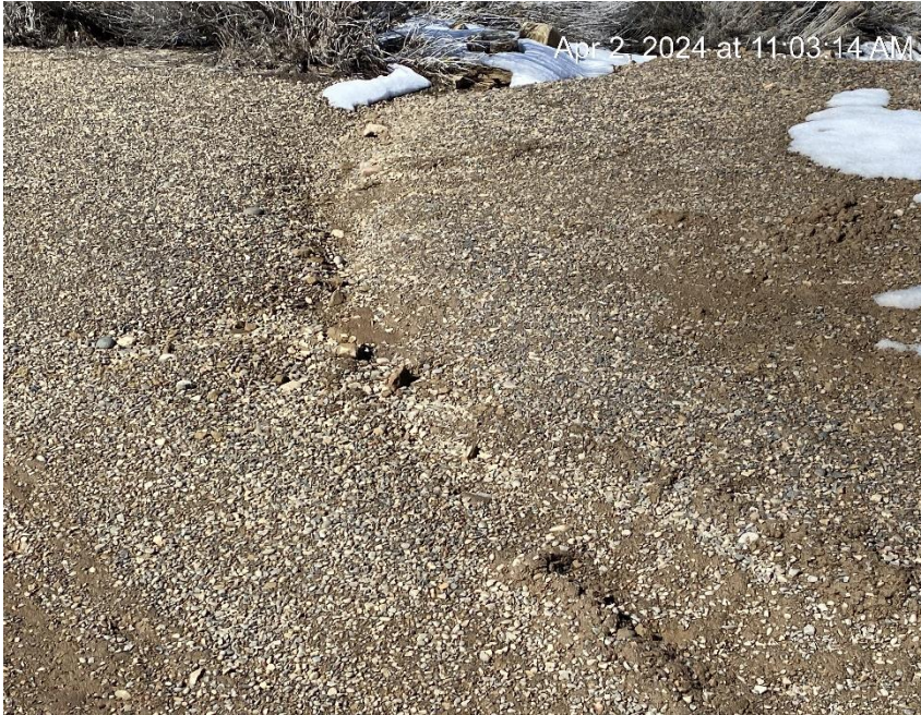
Erosion and sediment migration
