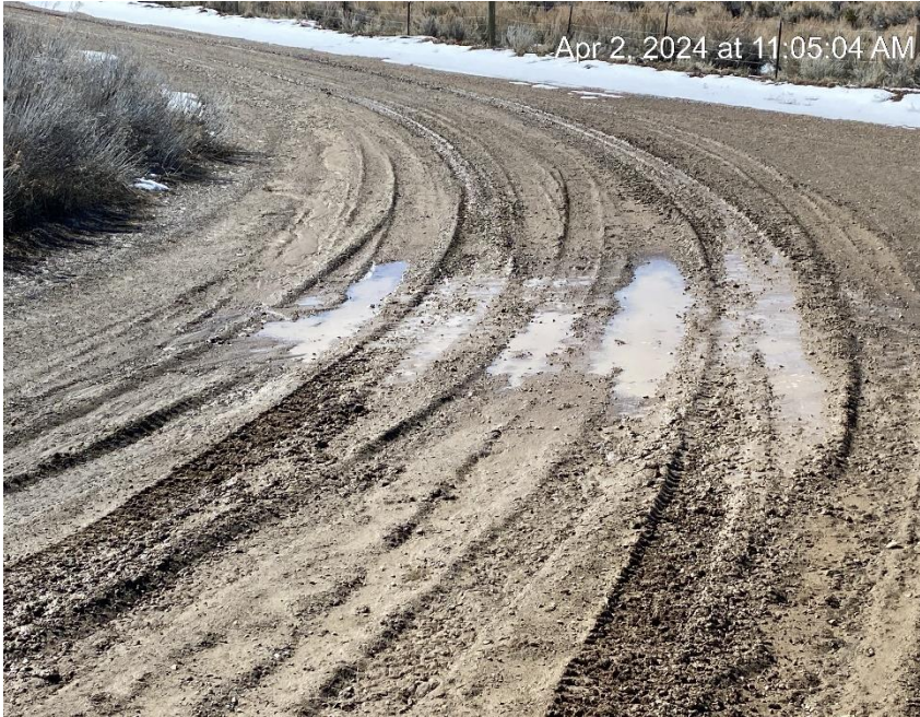
Sediment migration. Vehicle tracking from well pad.
