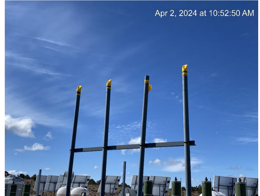
Relief riser missing rain protection
