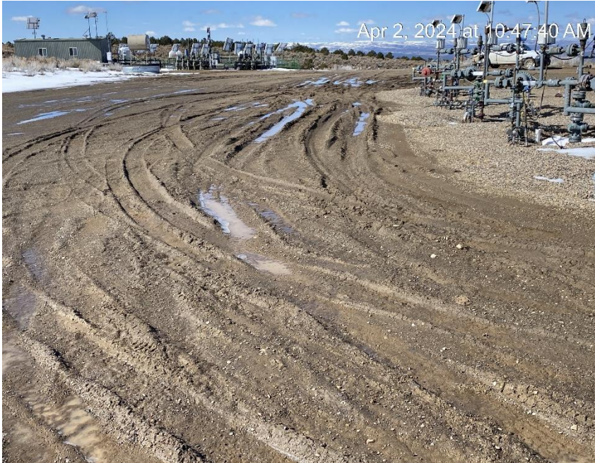
Lack of stabilization. Vehicle tracking.
