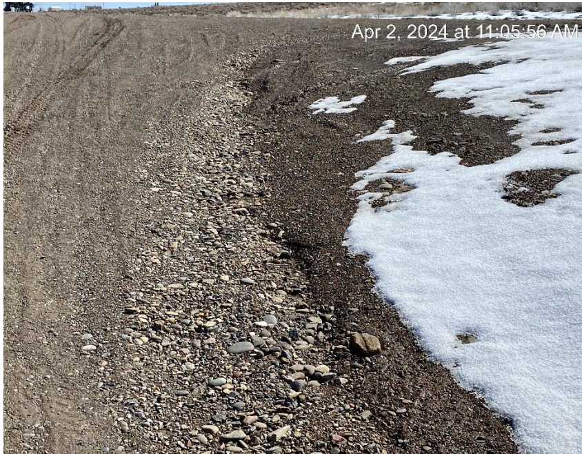
Erosion and sediment migration
