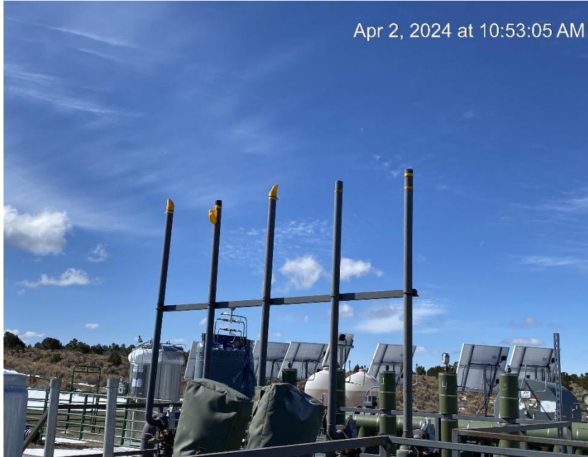
Relief risers missing rain protection
