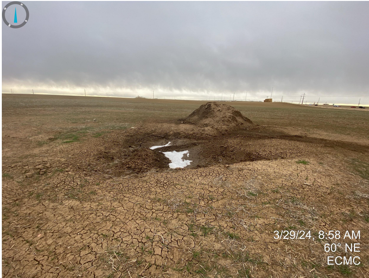
Photo 1. Location does not appear to have been graded/contoured to reflect adjacent lands. Open excavation observed at the time of this inspection.
