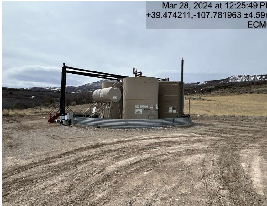
Location and Lack of stabilization/compaction
