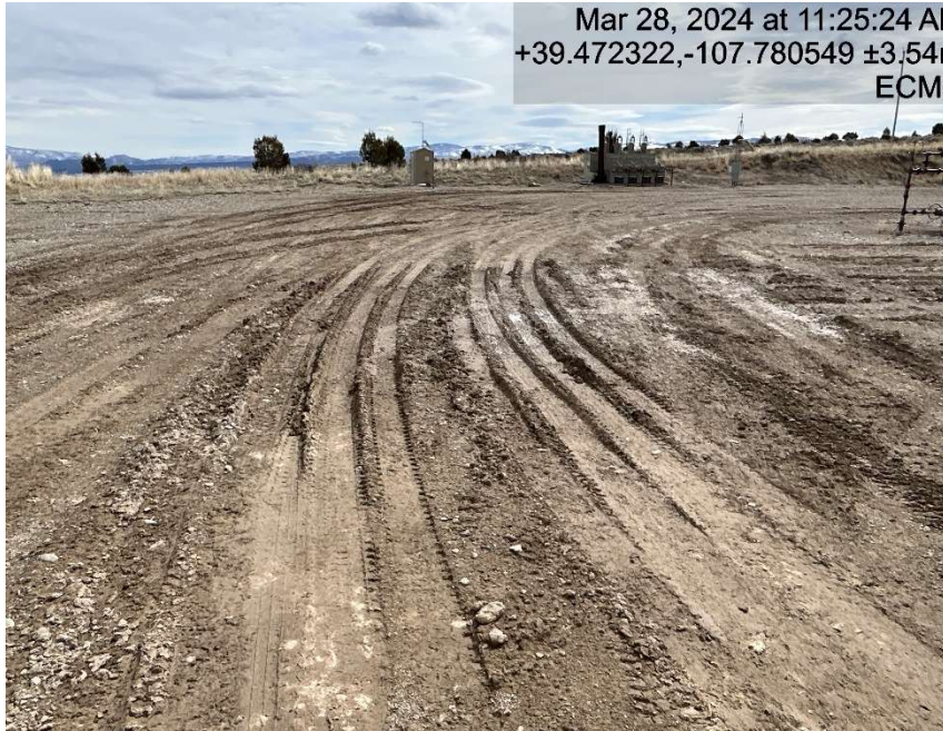
Lack of stabilization/compaction
