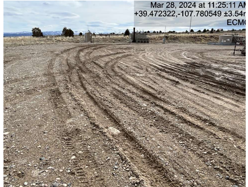
Lack of stabilization/compaction
