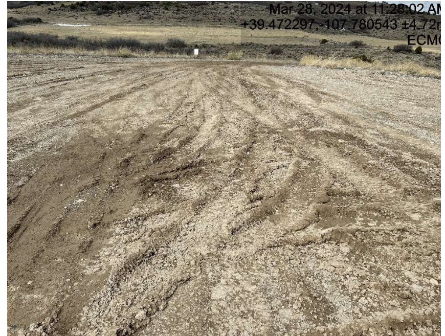
Lack of stabilization/compaction
