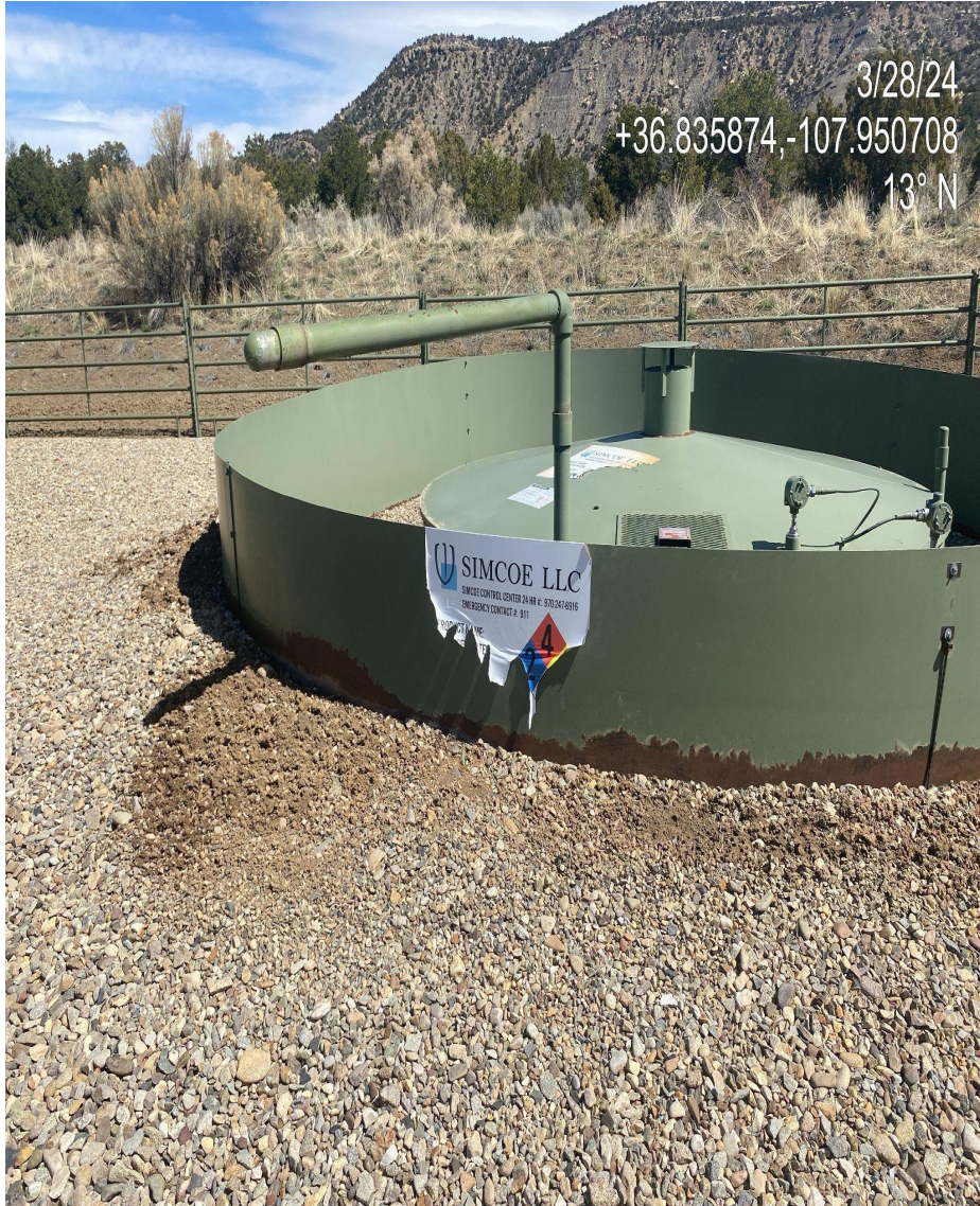
Photo 3. Both produced water signs/placards on location are deteriorating and no longer displaying tank capacity.
