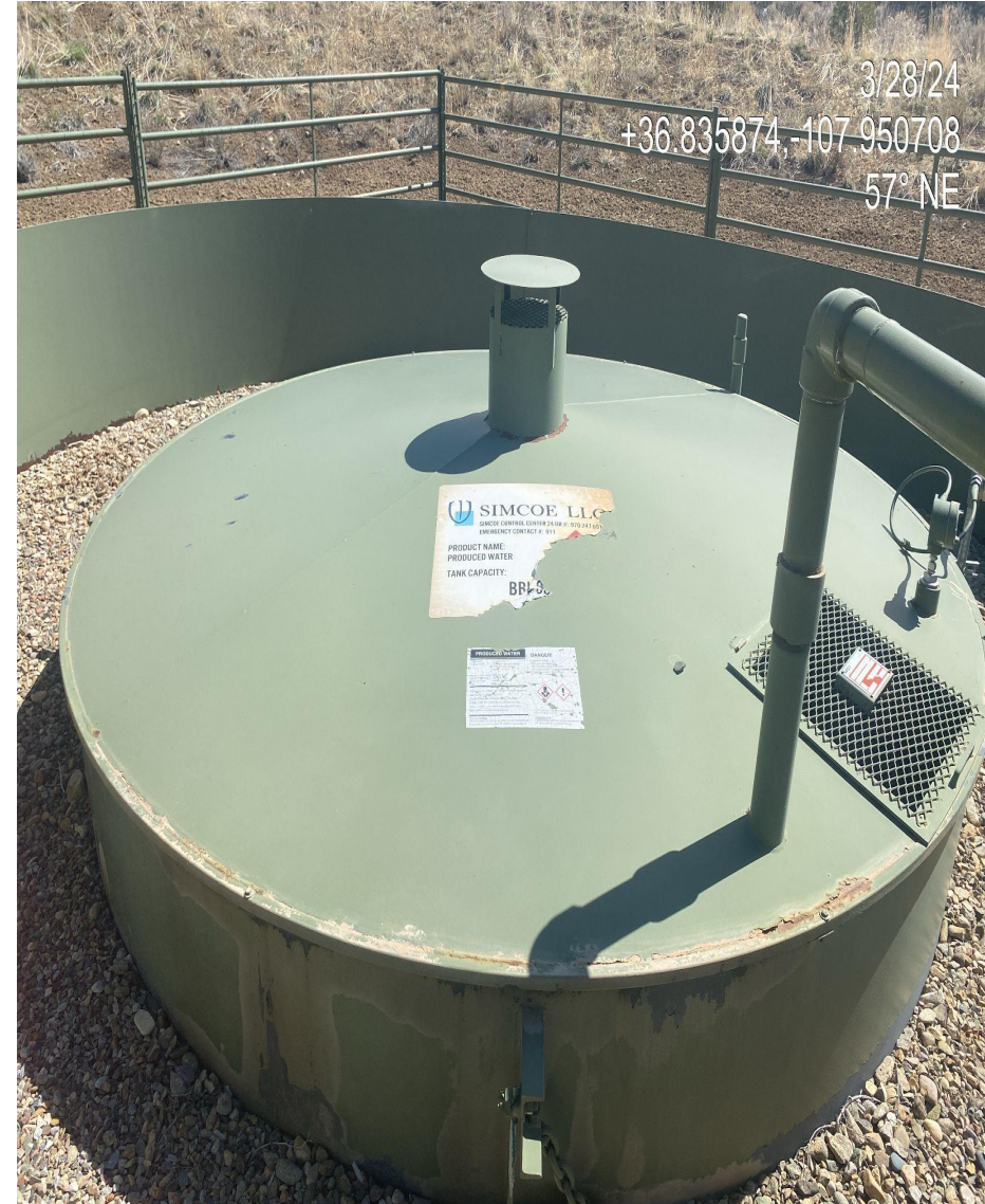
Photo 3. Both produced water signs/placards on location are deteriorating and no longer displaying tank capacity.
