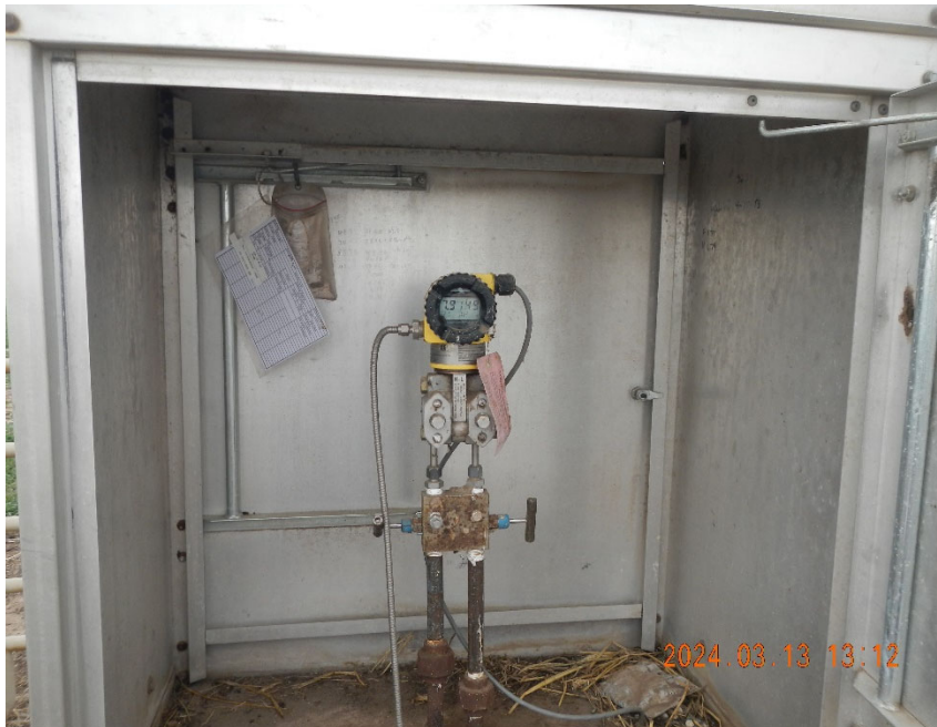
5. Digital meter inside meter box.
