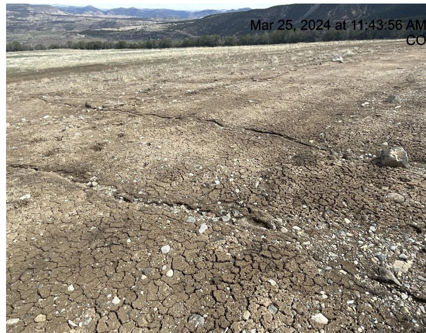
Photo # 1284 Rill erosion & transport of sediment off location/insufficient runoff controls/BMP's
