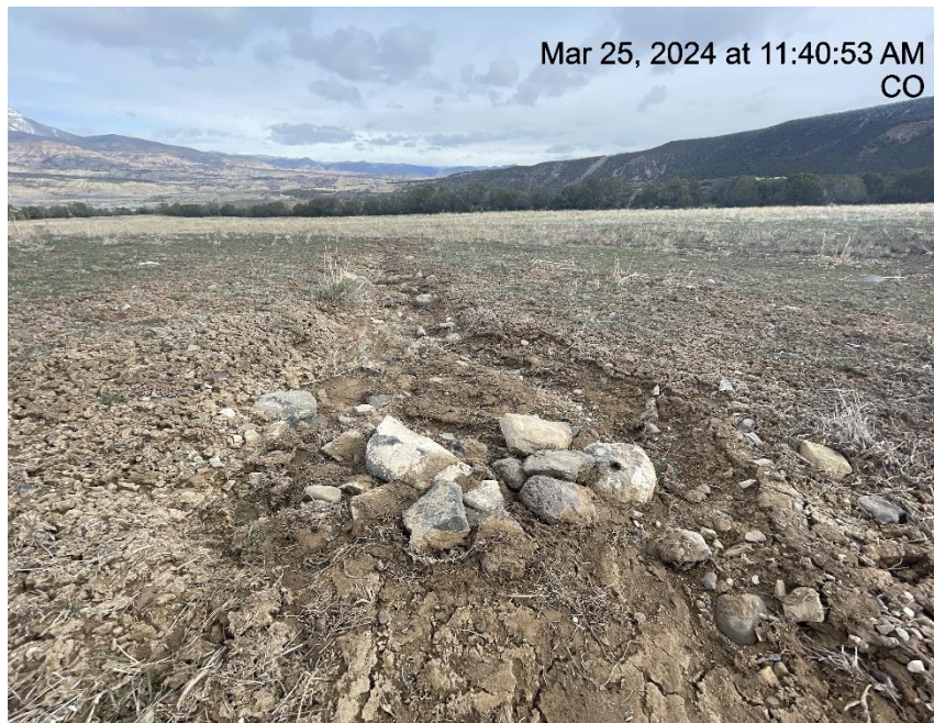
Photo # 1279 Check dam/BMP needs maintenance.
