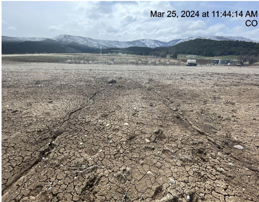
Photo # 1285 Rill erosion & transport of sediment off location/insufficient runoff controls/BMP's
