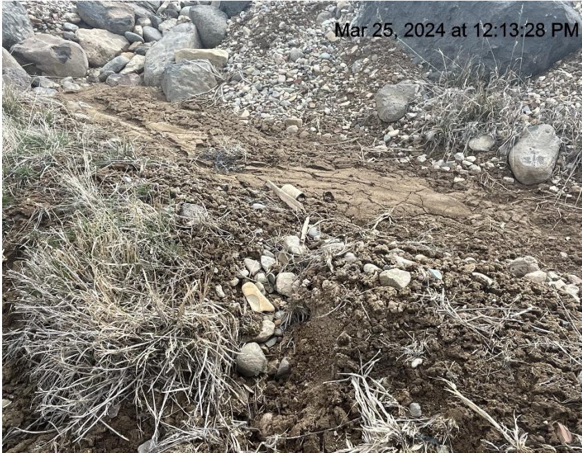
Photo # 1271 Ditch/BMP near entrance to location needs maintenance/sediment buildup & small breach in ditch allowing sediment transport from ditch into the interim area & causing more erosion & sediment transport in the interim area itself.
