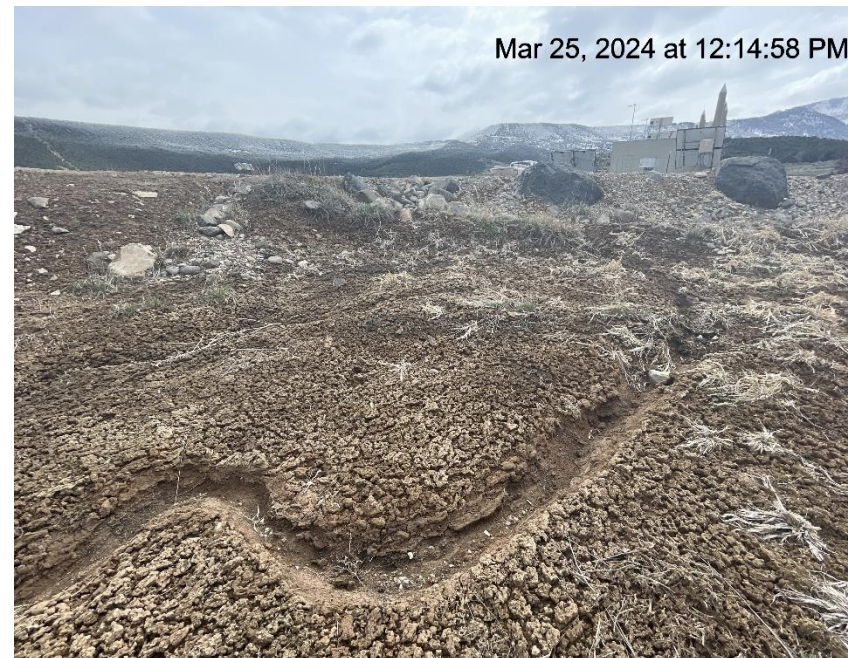
Photo # 1274 Ditch/BMP near entrance to location needs maintenance/small breach in ditch allowing sediment transport from ditch into the interim area & causing more erosion & sediment transport in the interim area itself.
