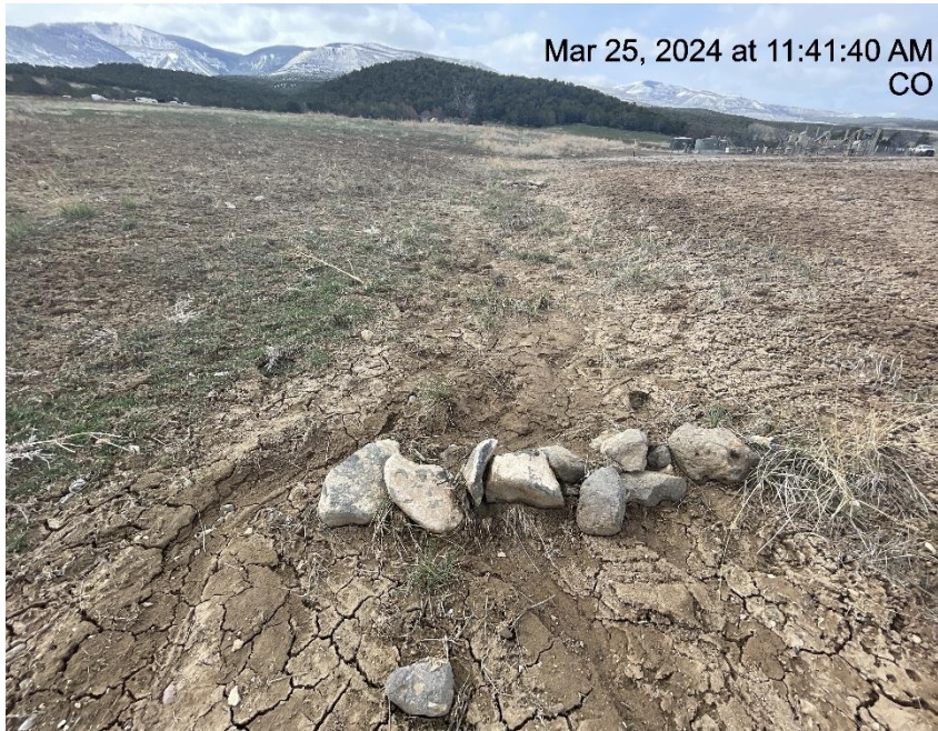
Photo # 1281 Check dam/BMP needs maintenance.
