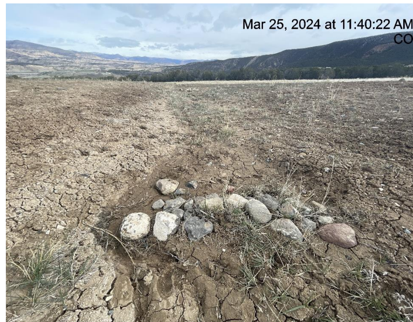
Photo # 1276 Check dam/BMP needs maintenance.
