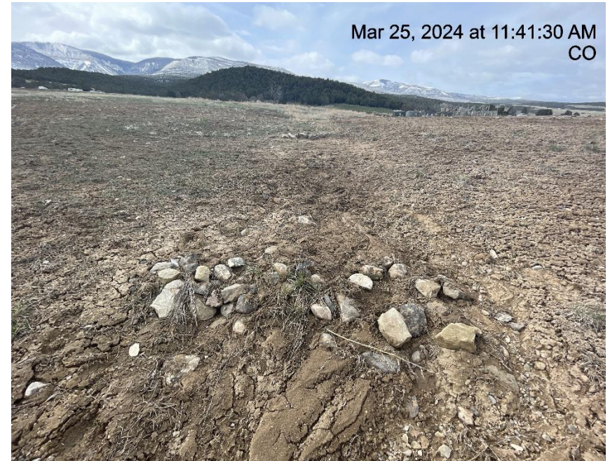
Photo # 1282 Check dam/BMP needs maintenance.
