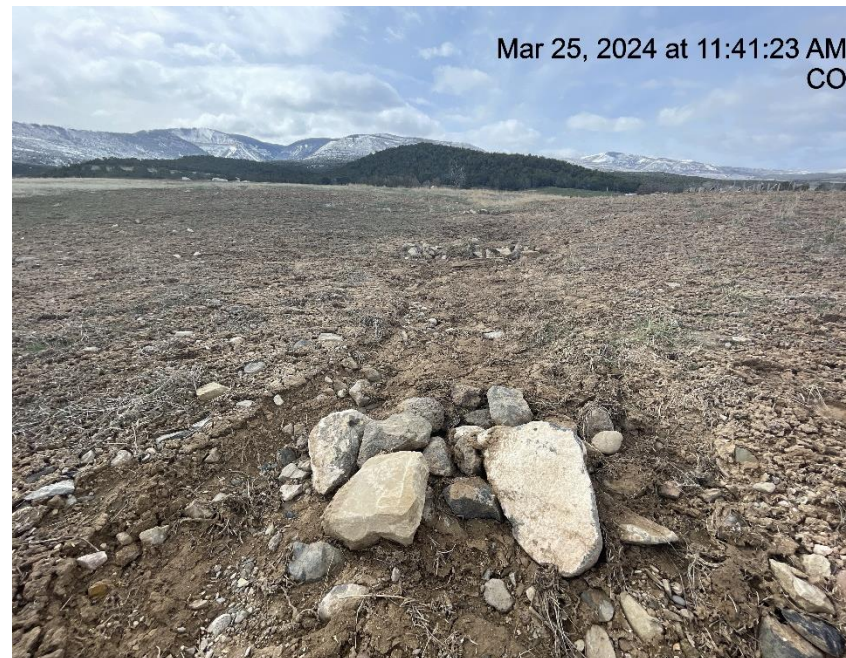
Photo # 1280 Check dam/BMP needs maintenance.
