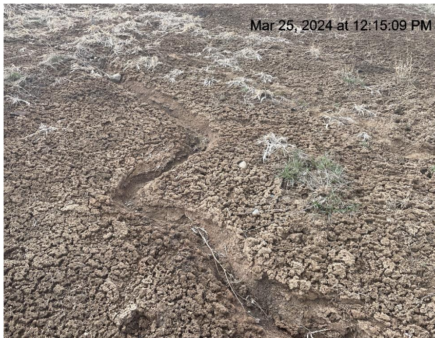
Photo # 1275 Ditch/BMP near entrance to location needs maintenance/small breach in ditch allowing sediment transport from ditch into the interim area & causing more erosion & sediment transport in the interim area itself.
