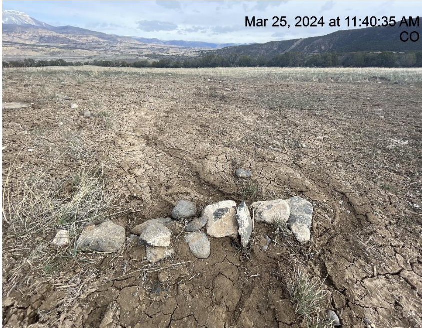
Photo # 1277 Check dam/BMP needs maintenance.
