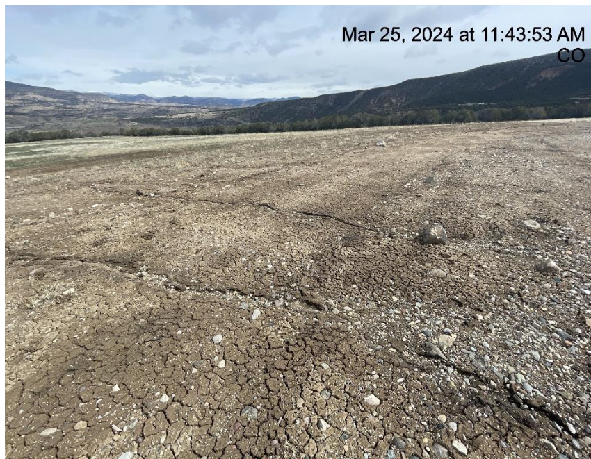
Photo # 1283 Rill erosion & transport of sediment off location/insufficient runoff controls/BMP's
