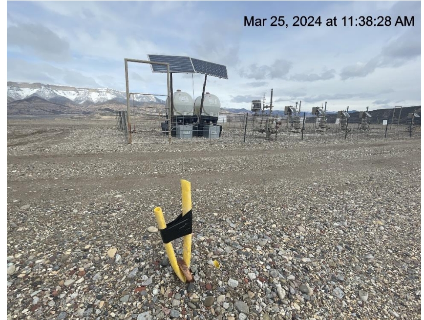
Photo # 1269 Improperly marked deadman
