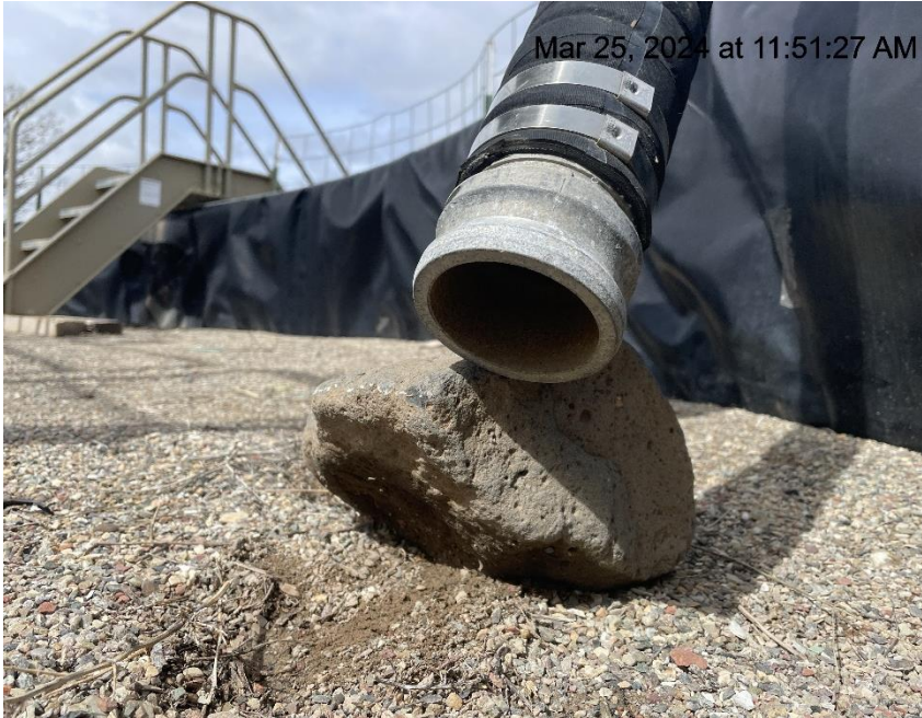
Photo # 1268 Hose on pump open ended/wildlife hazard
