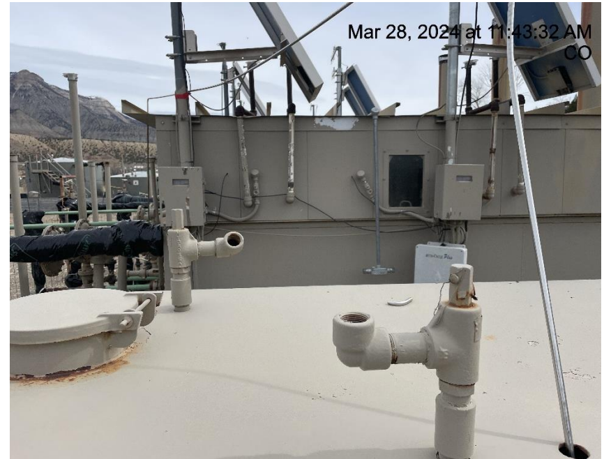
Photo # 1731 PRV's do not comply with CECMC pressure safety device rules.
