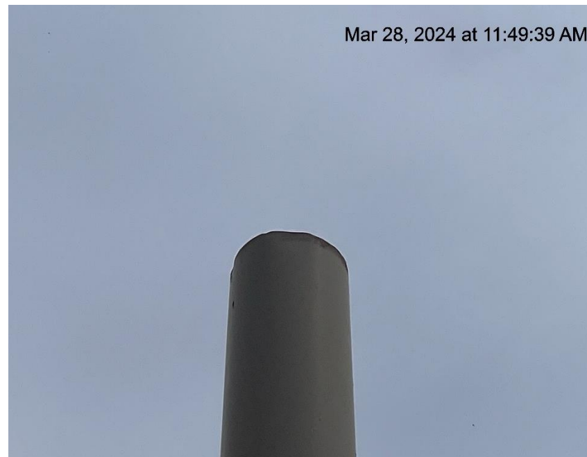
Photo # 1733 Separator burner exhaust stack lacks bird protection/does not comply with CECMC wildlife rules.
