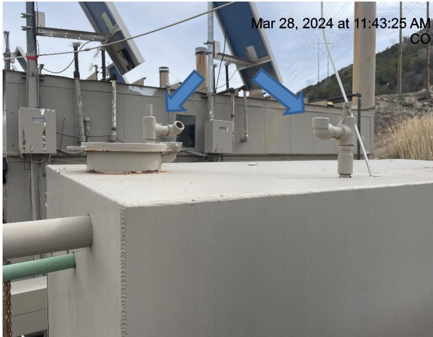
Photo # 1730 PRV's do not comply with CECMC pressure safety device rules.
