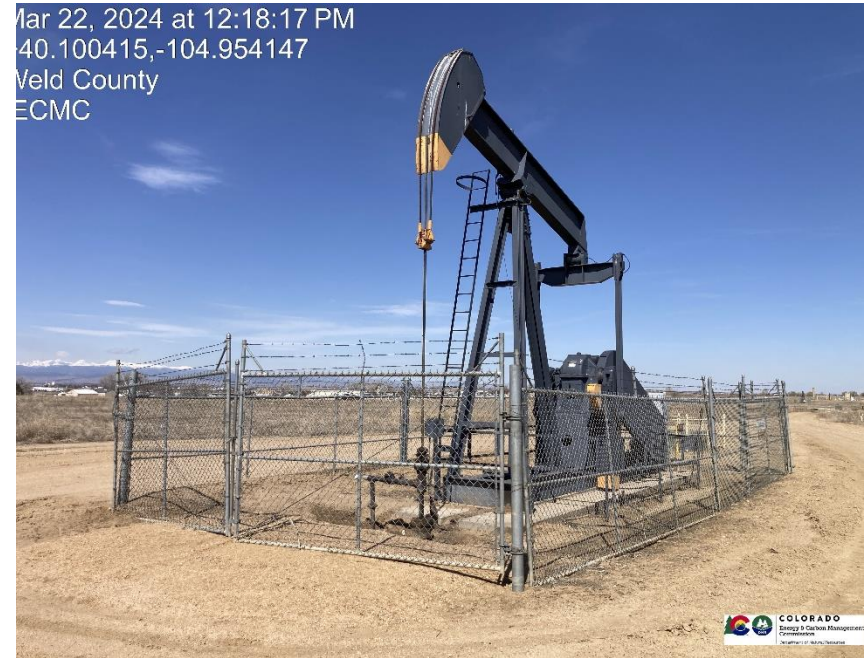
Pic 2 pupm jack / wellhead
