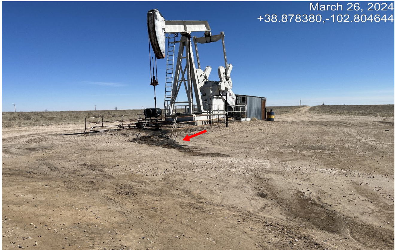
Photo 3. Facing northeast toward the wellsite. There is oil leaking out of the wellhead that must be controlled and cleaned up.
