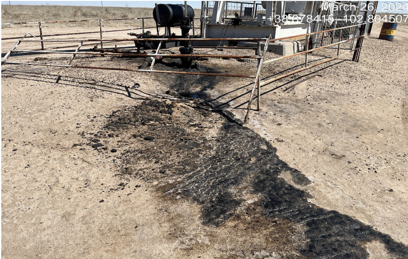
Photo 4. View of oil that has leaked out of the well.
