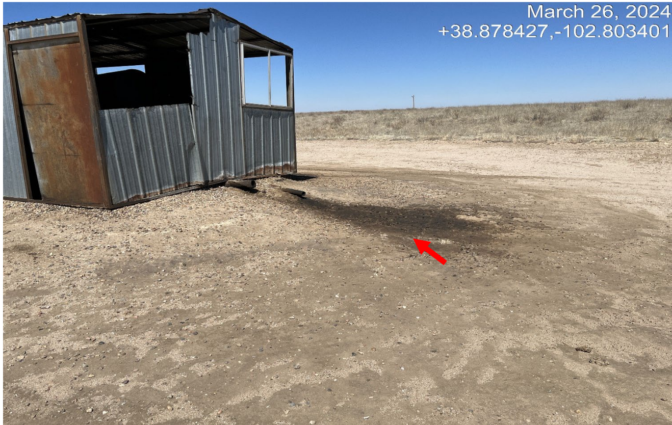
Photo 5. There is oil coming out of the exhaust pipe which is staining the soil and needs to be cleaned up.
