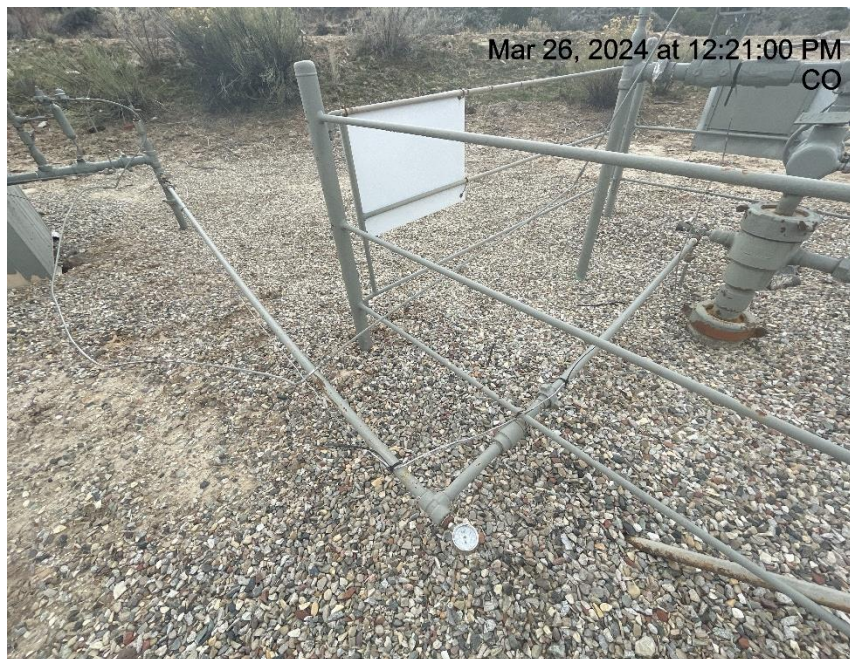
Photo # 1534 KNIGHT W-6-4 bradenhead tied into flowline/No Form 4 Sundry
