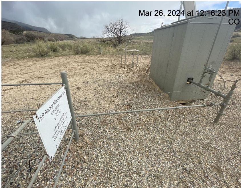
Photo # 1536 KNIGHT W-6-4 bradenhead tied into flowline/No Form 4 Sundry
