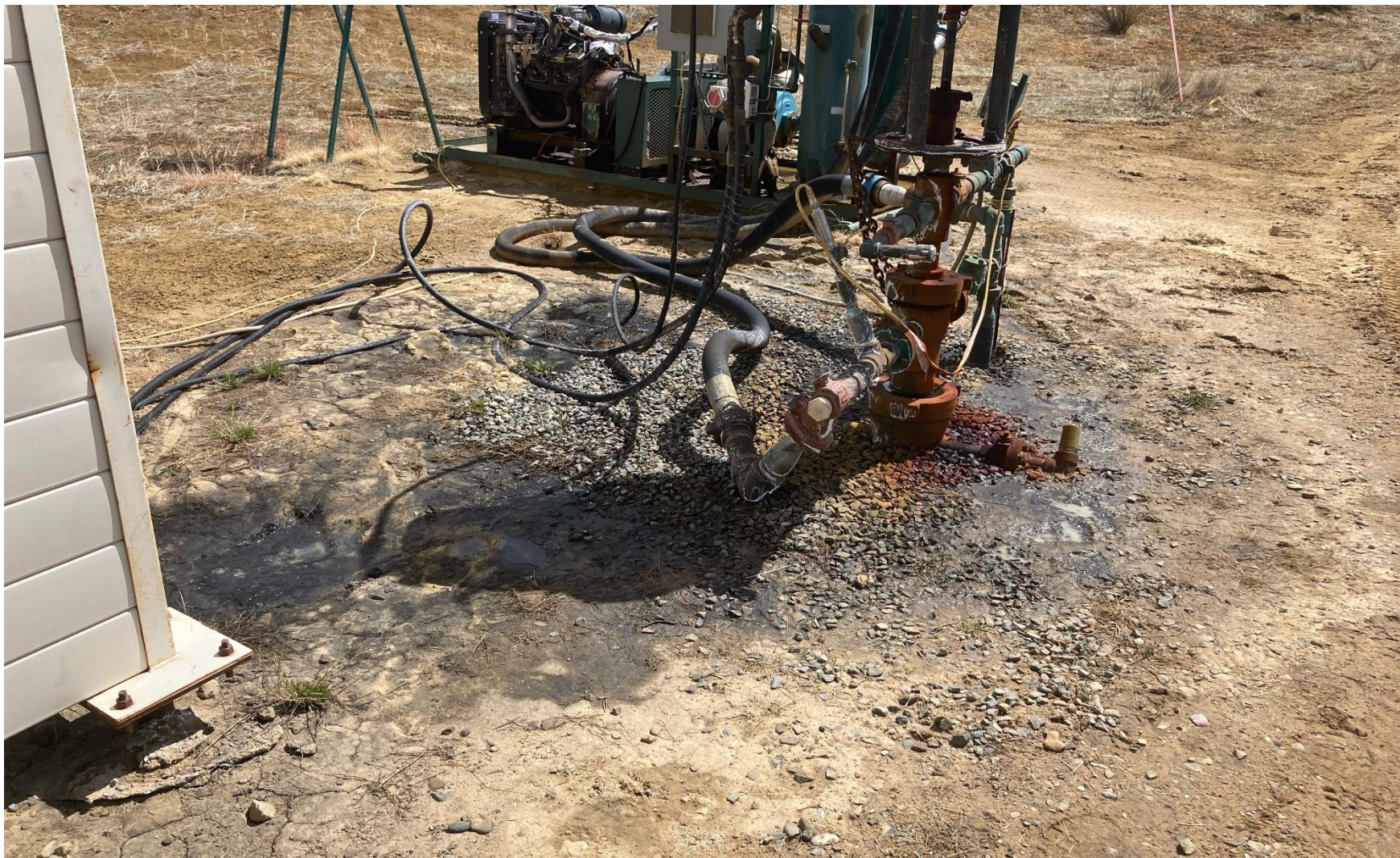
PHOTO 4: Signs of recent slow leak from wellhead has left a Salt/black mineral buildup around the wellhead. Securely fasten all valves, pipes, fittings, and Production Facilities to ensure good mechanical condition, inspect at regular intervals and maintain in good mechanical condition remove and dispose of impacted material per Rule 608.e. ca date 4-27-2024.
