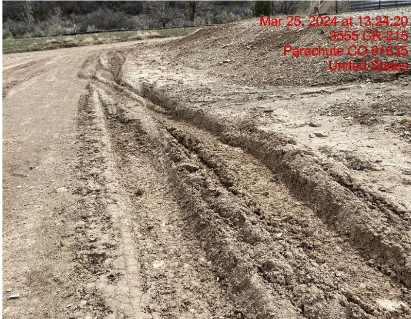
Lack of Stabilization – Photo #00050
