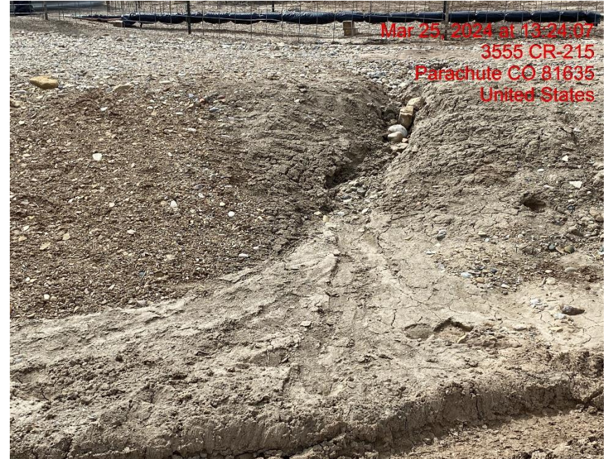
Insufficient Erosion Control – Photo #00049
