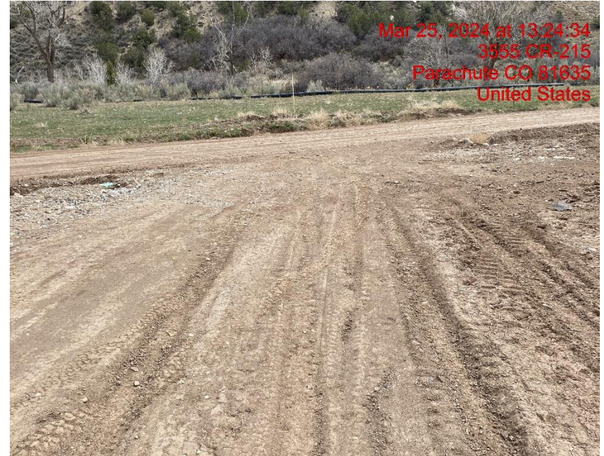
Insufficient Vehicle Tracking BMPs at Location Entrance/Exit – Photo #00051
