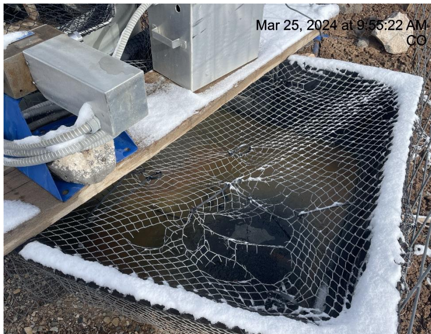
Photo # 1143 Netting/wildlife protection needs maintenance
