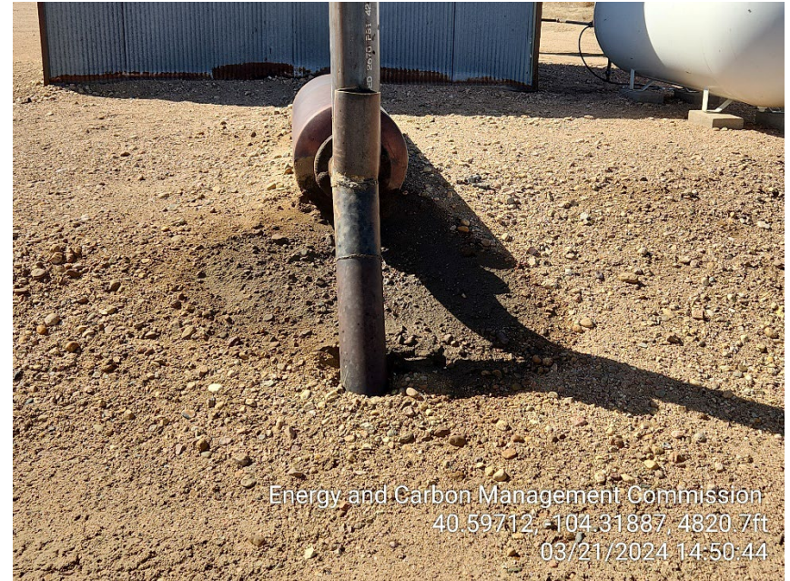
Photo 2 – Stained Soil at Exhaust
