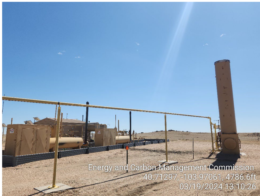
Photo 5 – Separators and ECD
