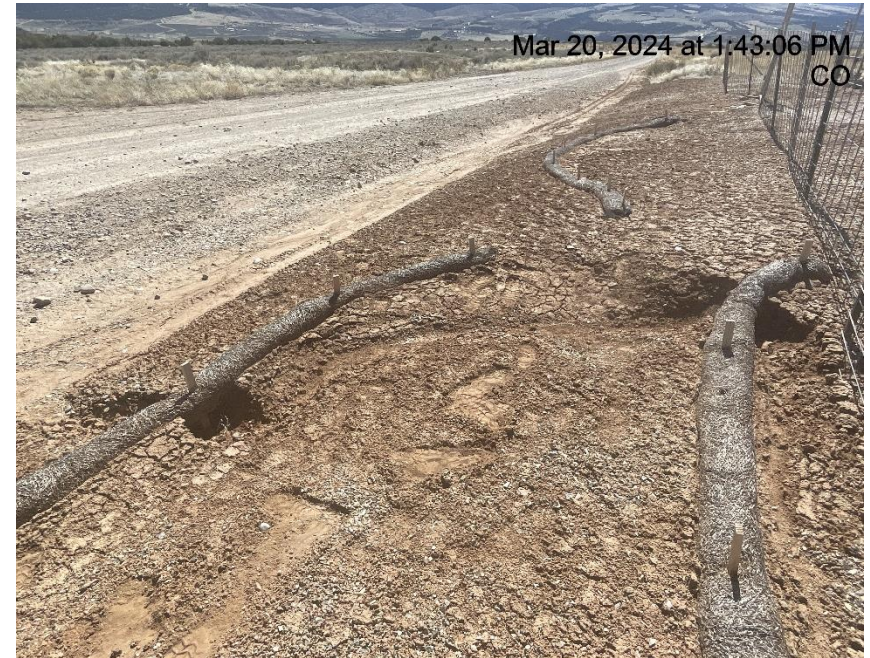
Photo # 782 Wattles need maintenance/stormwater undercutting BMP's & transporting sediment off location
