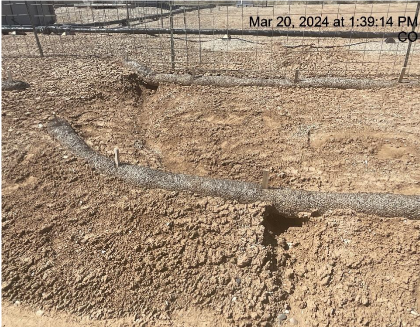
Photo # 783 Wattles need maintenance/stormwater undercutting BMP's & transporting sediment off location
