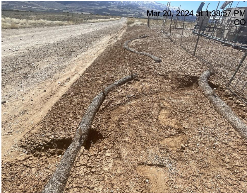
Photo # 781 Wattles need maintenance/stormwater undercutting BMP's & transporting sediment off location
