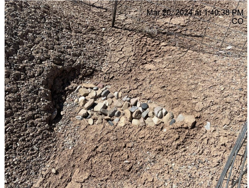
Photo # 784 Check dam needs maintenance/stormwater eroding around BMP & cutting into secondary containment berm
