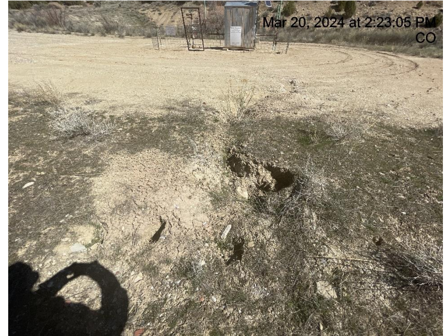
Photo # 830 Erosion & transport of sediment off location & into a vegetated area
