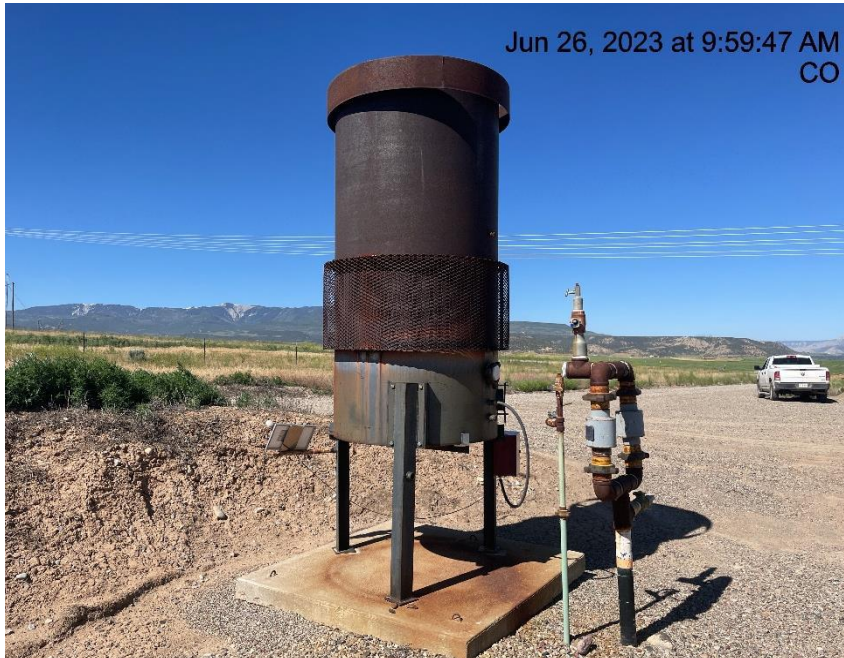
Photo # 1802 from inspection 708900877 conducted on 06/26/2023 - Unused equipment/ECD disconnected
