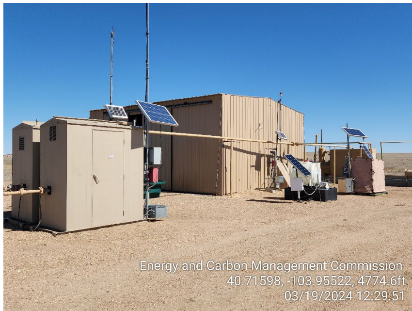
Photo 3 – Compressor, Gas Meters and VRU
