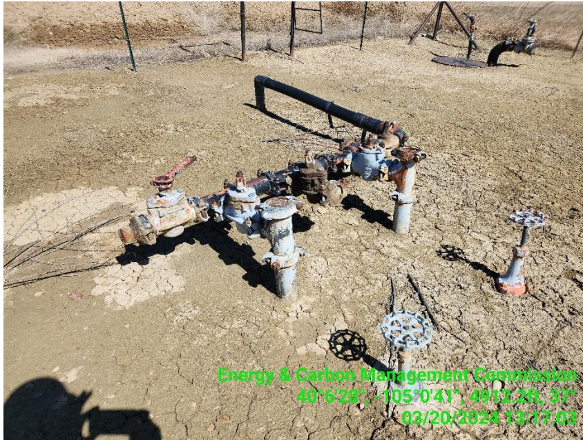
Photo 11 Flow line manifold west of the wellsite.
