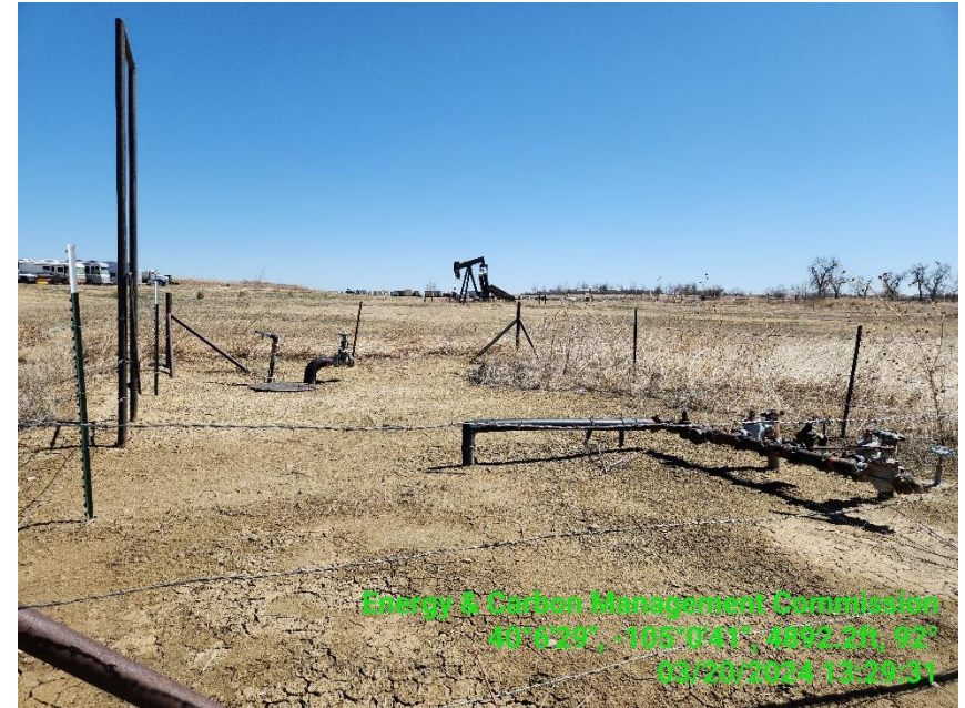
Photo 12 Flow line manifold west of the wellsite.
