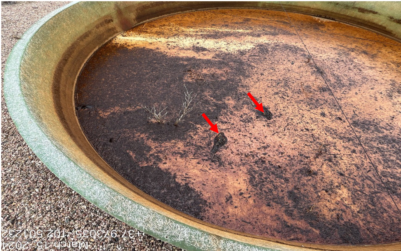
Photo 5. There is no wildlife protection on the open top tank. Red arrows point to dead birds found in the tank.
