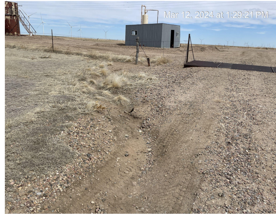
Photo 8. Photo taken facing east of stormwater erosion on access road leading from tank battery to well pad.
