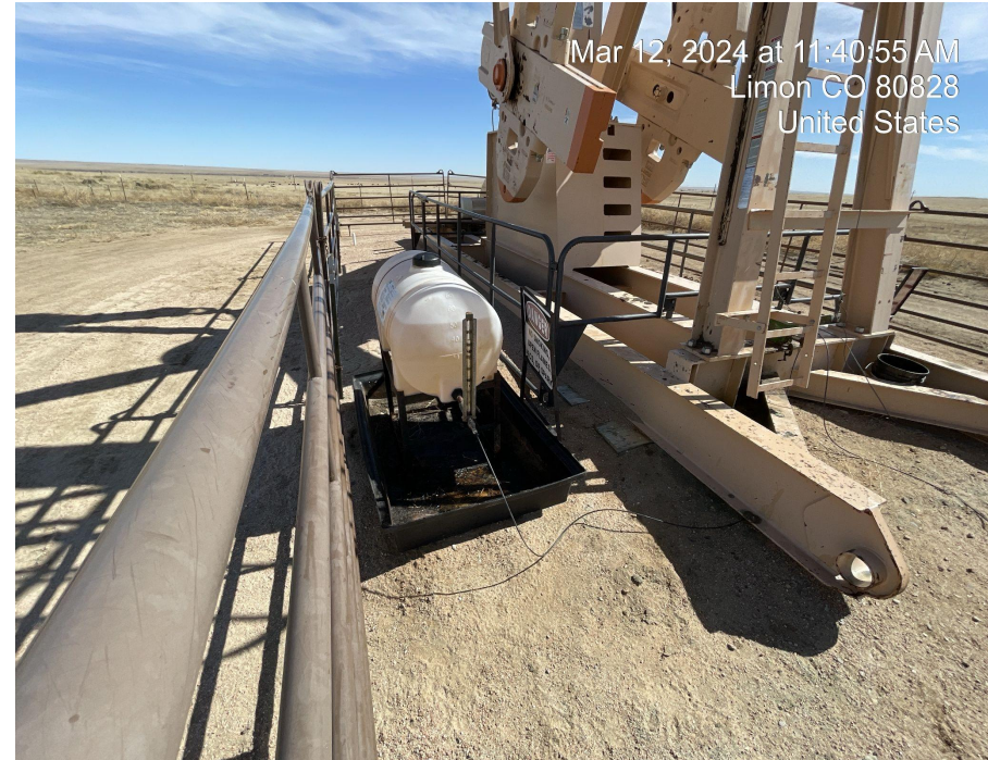
Photo 4. Photo taken facing east of secondary containment without wildlife protection.
