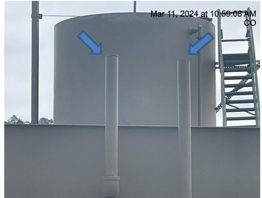
Photo # 9148 PRV & rupture disc vent lines lack caps/do not comply with CECMC pressure safety device rules
