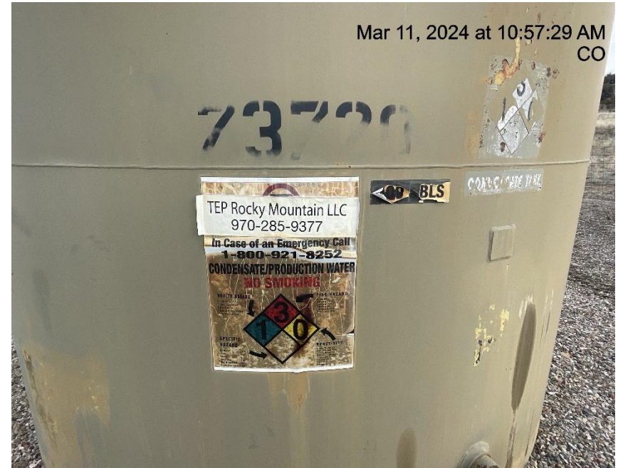
Photo # 9146 Tank label damaged & some required information is illegible
