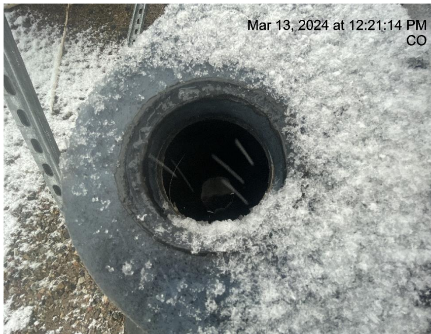
Photo # 9779 Chemical containment approximately \frac{3}{4} full of fluid/Failure to maintain chemical BMP/BMP insufficient to contain possible spill
