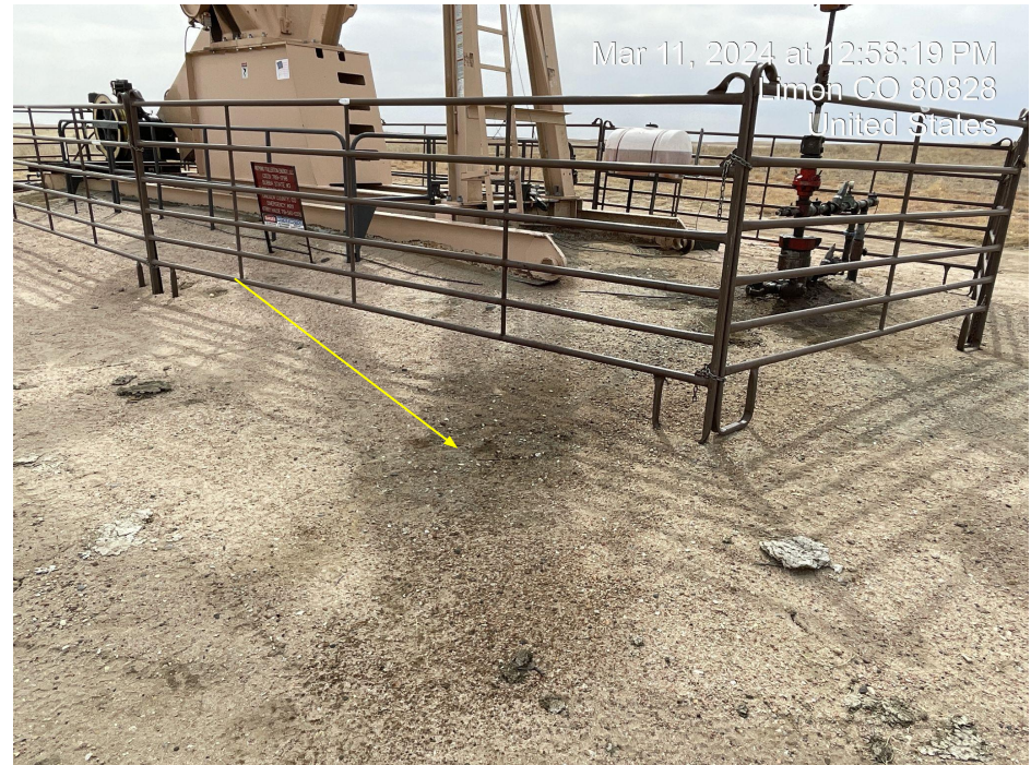
Photo 4. Photo taken facing southeast of staining around wellhead. yellow arrow indicates staining outside fenced area.
