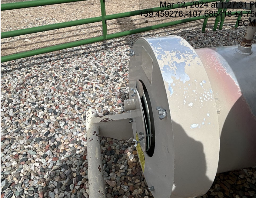
Burner assembly is propped open bypassing the spark arrester
