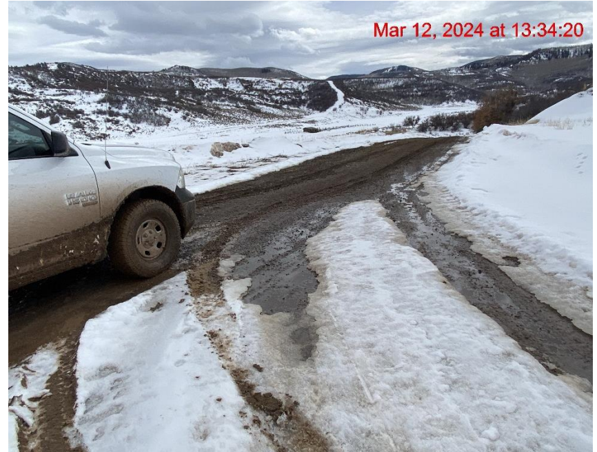
Insufficient Vehicle Tracking BMPs at Location Entrance/Exit – Photo #09881
