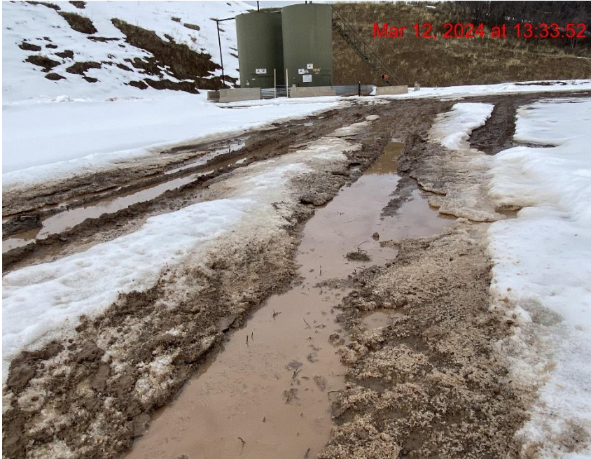
Lack of Stabilization – Photo #09880
