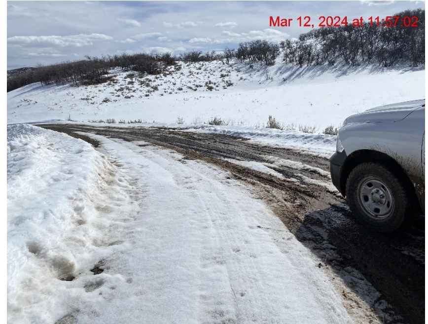
Insufficient Vehicle Tracking BMPs at Location Entrance/Exit – Photo #09827
