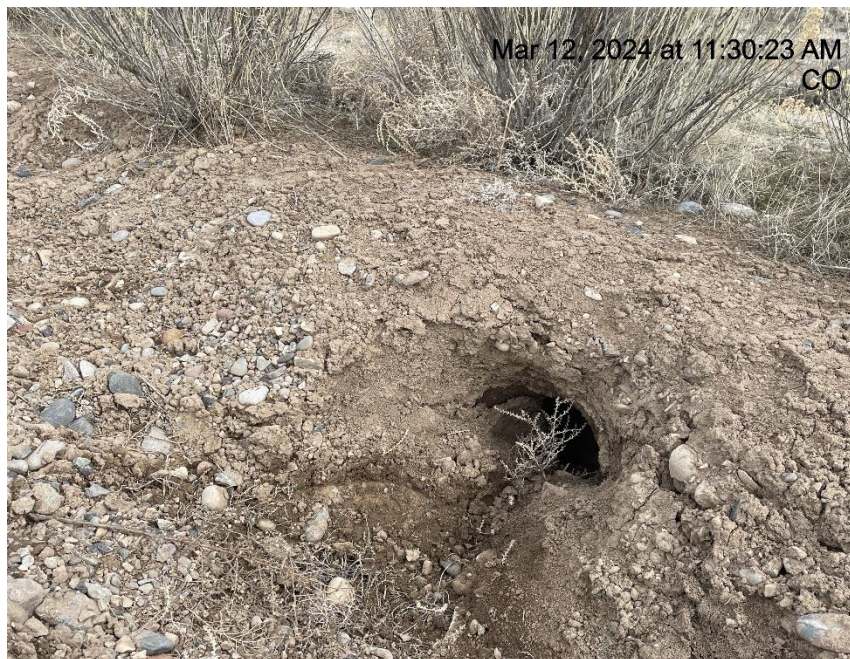
Photo # 9428 Tunnel erosion through berm/berm needs maintenance (N/NE area of location)
