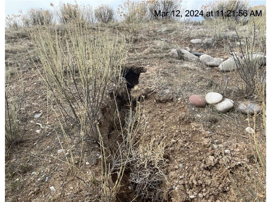
Photo # 9431 Tunnel erosion through berm/erosion & transport of sediment off location (N/NE area on opposite side of berm just off location)
