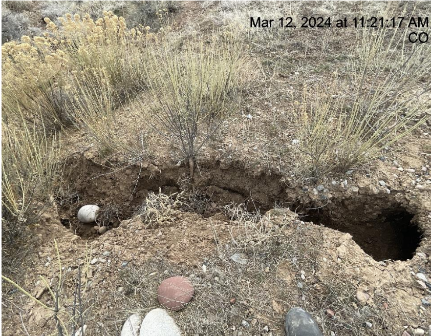
Photo # 9430 Tunnel erosion through berm/erosion & transport of sediment off location (N/NE area on opposite side of berm just off location)
