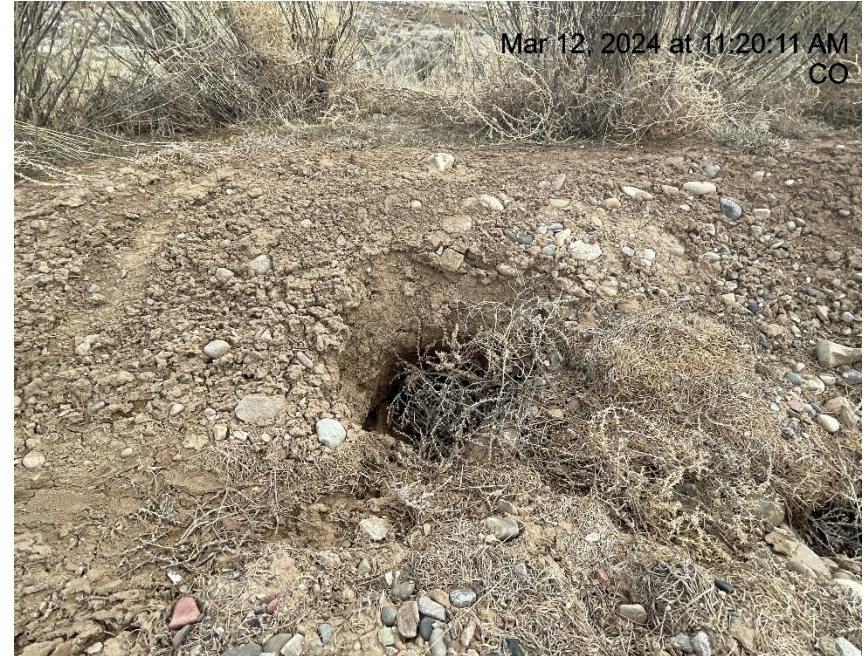
Photo # 9433 Tunnel erosion through berm/berm needs maintenance (N/NE area of location)
