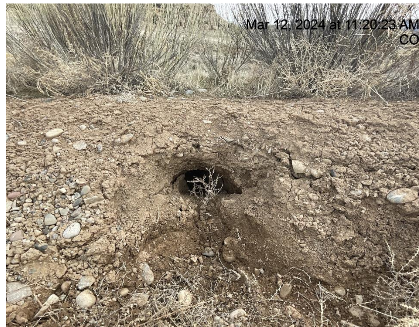
Photo # 9429 Tunnel erosion through berm/berm needs maintenance (N/NE area of location)
