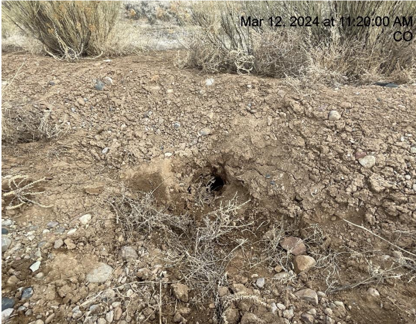
Photo # 9432 Tunnel erosion through berm/berm needs maintenance (N/NE area of location)
