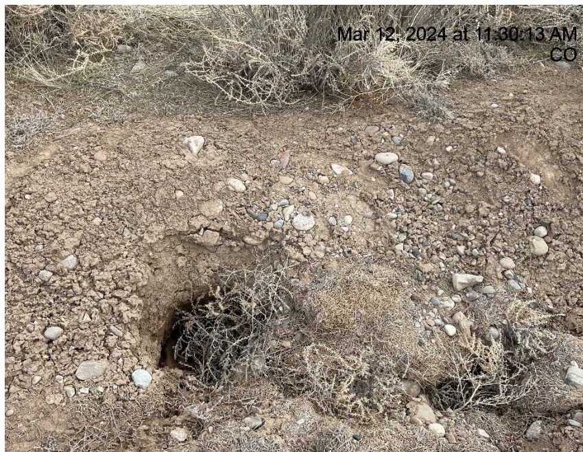
Photo # 9434 Tunnel erosion through berm/berm needs maintenance (N/NE area of location)
