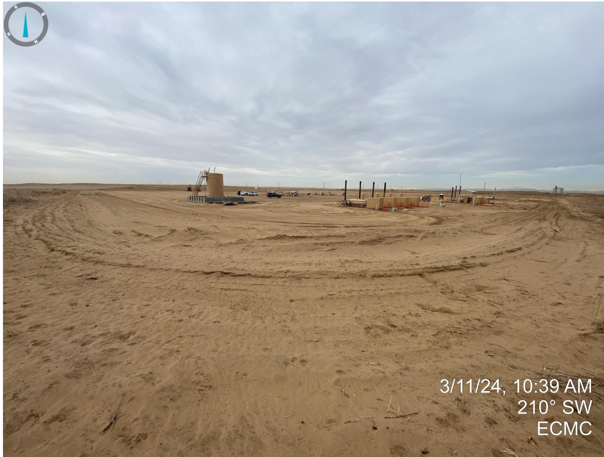
Photo 7. Northeast corner of location. Perimeter stormwater control (ditch and berm) has been constructed around the location. Soils appear to be unstabilized and require additional stabilization BMPs.
