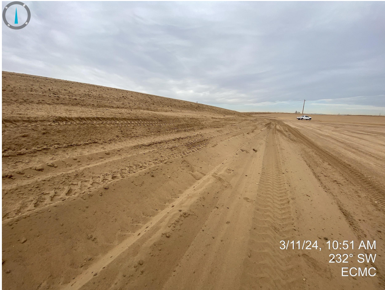
Photo 14. North side of topsoil stockpile. The stockpile does not appear to be properly stabilized from wind/water erosion with evidence of unstabilized soils. Temporary BMPs (e.g. equipment tracking) should be implemented prior to selecting more permanent BMPs.
