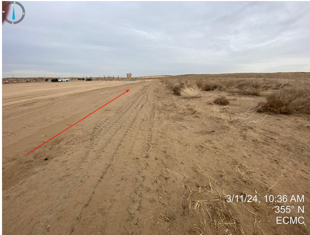
Photo 6. East side of location. Perimeter stormwater control (ditch and berm) has been constructed around the location. Soils appear to be unstabilized and require additional stabilization BMPs.
