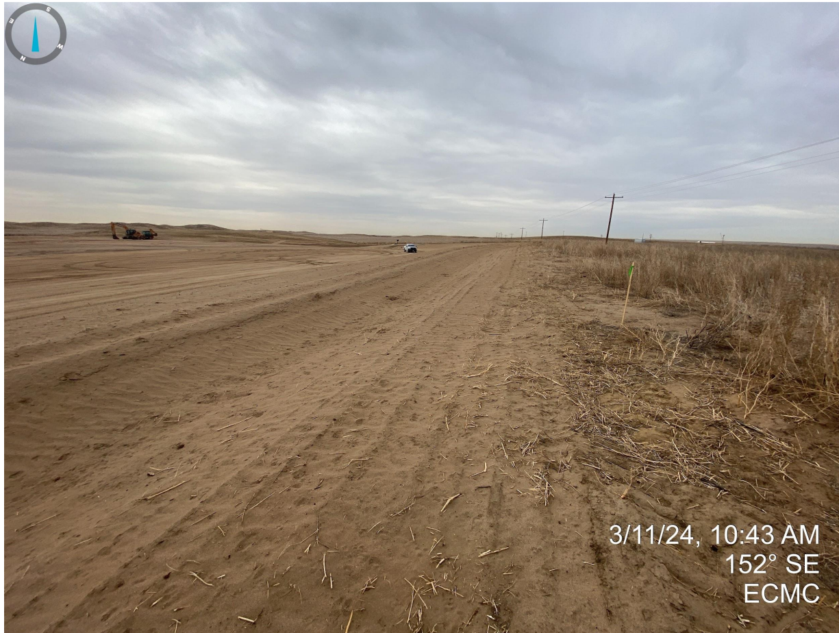
Photo 9. West side of location. Perimeter stormwater control (ditch and berm) has been constructed around the location. Soils appear to be unstabilized and require additional stabilization BMPs.
