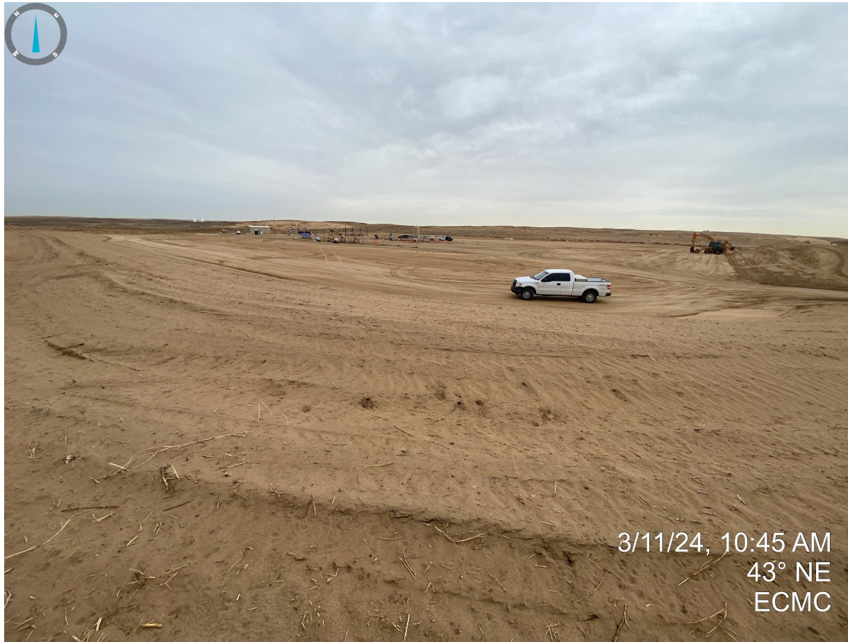
Photo 10. Southwest corner of location. Perimeter stormwater control (ditch and berm) has been constructed around the location. Soils appear to be unstabilized and require additional stabilization BMPs.
