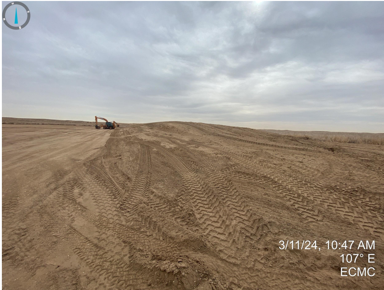
Photo 11. West side of topsoil stockpile. The stockpile does not appear to be properly stabilized from wind/water erosion with evidence of unstabilized soils. Temporary BMPs (e.g. equipment tracking) should be implemented prior to selecting more permanent BMPs.
