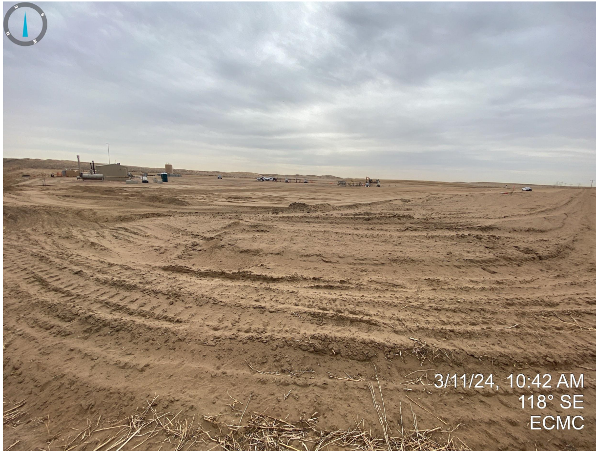
Photo 8. Northwest corner of location. Perimeter stormwater control (ditch and berm) has been constructed around the location. Soils appear to be unstabilized and require additional stabilization BMPs.
