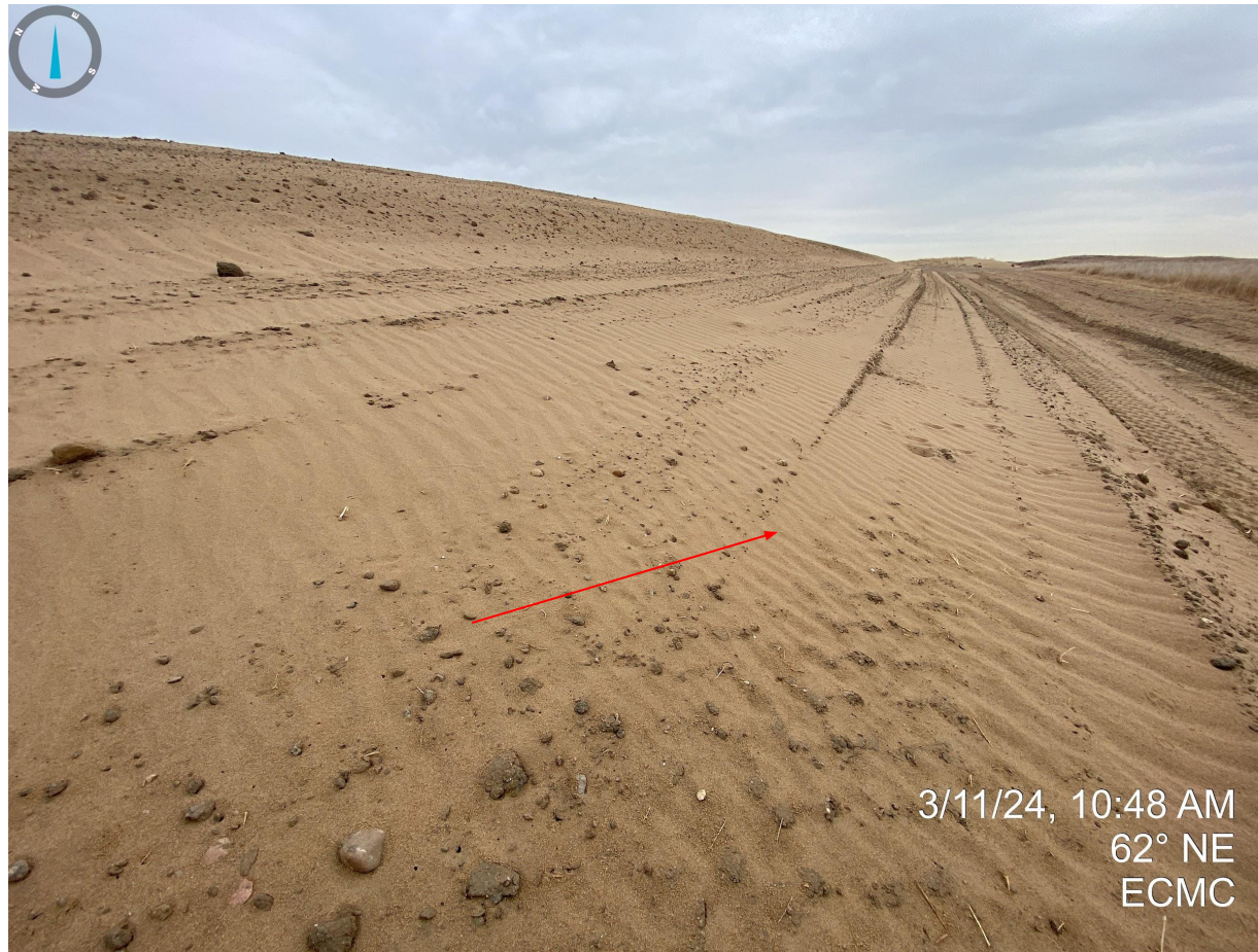
Photo 12. South side of topsoil stockpile. The stockpile does not appear to be properly stabilized from wind/water erosion with evidence of unstabilized soils. Temporary BMPs (e.g. equipment tracking) should be implemented prior to selecting more permanent BMPs. Red arrow indicates an example of wind erosion.
