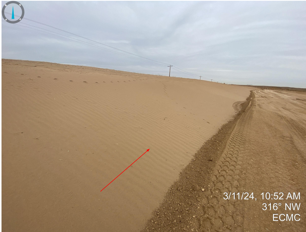
Photo 15. West side of location. The cut slopes do not appear to be properly stabilized from wind/water erosion with evidence of unstabilized soils. Temporary BMPs (e.g. equipment tracking) should be implemented prior to selecting more permanent BMPs. Evidence of wind erosion indicated by red arrow.
