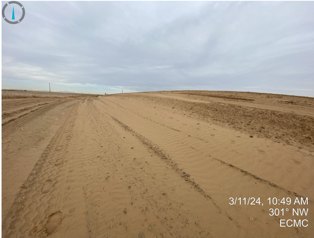
Photo 13. East/south side of topsoil stockpile. The stockpile does not appear to be properly stabilized from wind/water erosion with evidence of unstabilized soils. Temporary BMPs (e.g. equipment tracking) should be implemented prior to selecting more permanent BMPs.
