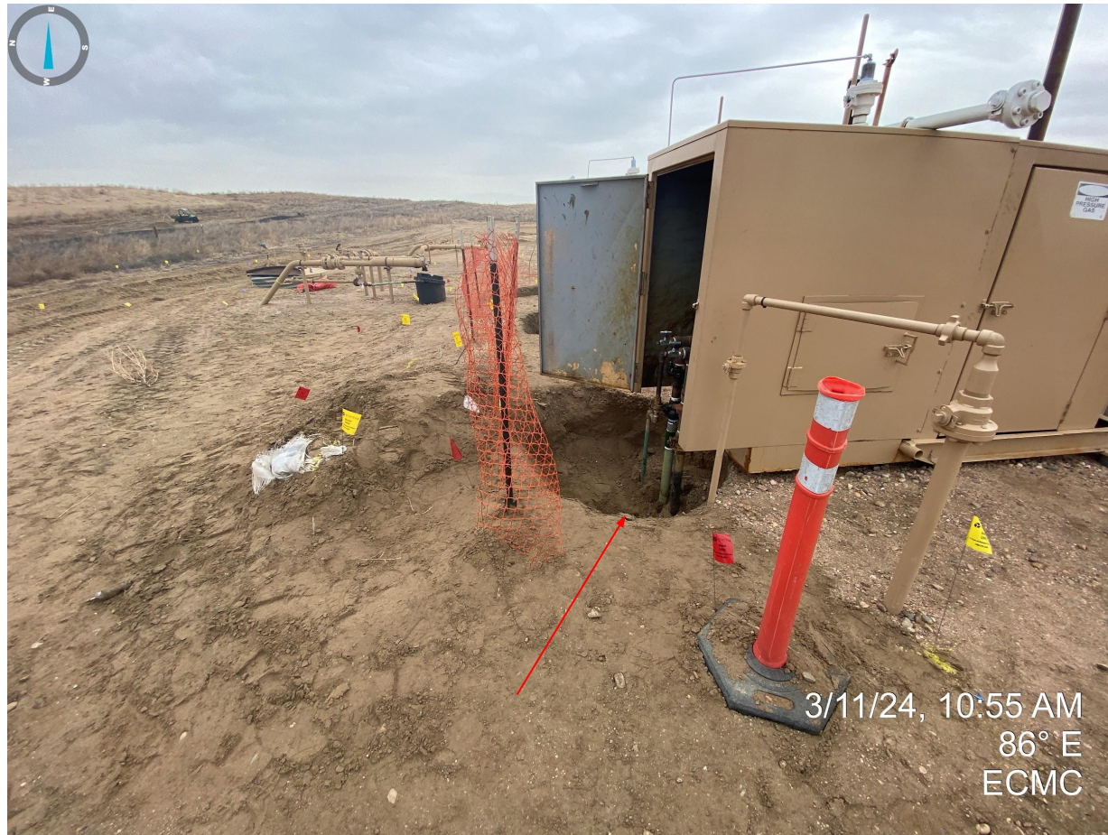
Photo 16. North side of location. Open excavations are not adequately fenced to exclude wildlife and/or people. Operator shall ensure that all open excavations are properly fenced when the location is unattended.
