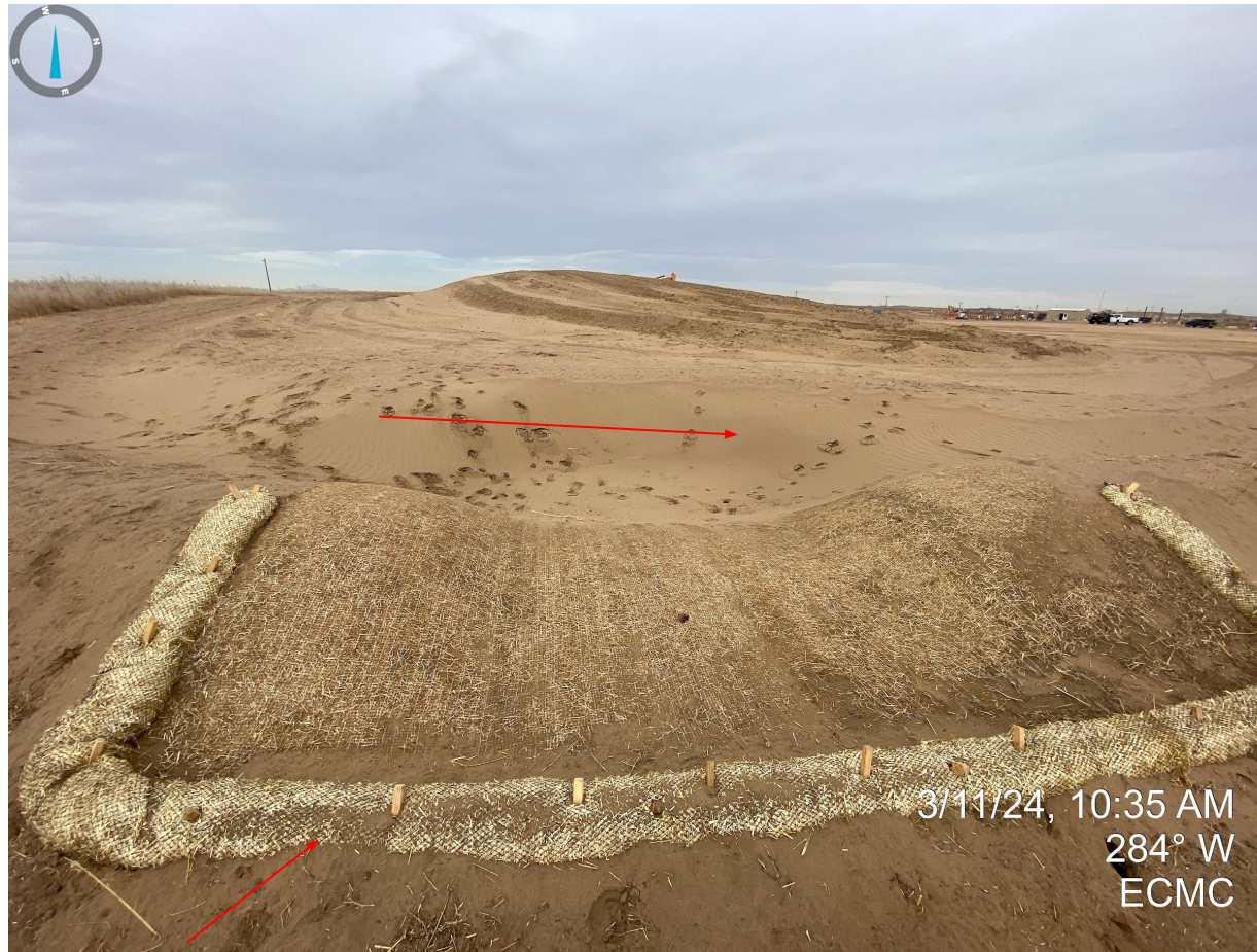
Photo 4. Continued form Photo 3. Red arrow indicates blow sand deposition from the unstabilized areas.
