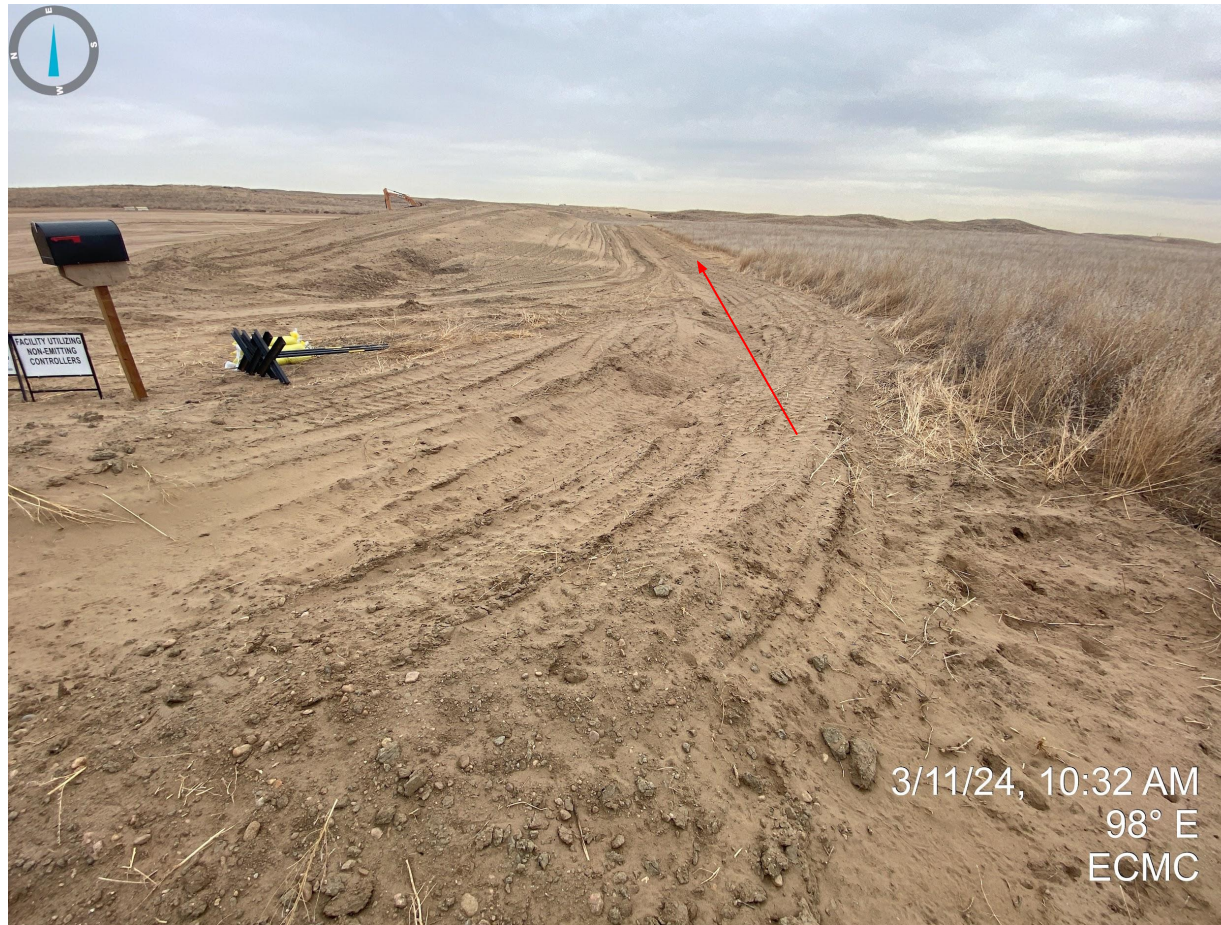
Photo 2. South side of location, near entrance. Perimeter stormwater control (ditch and berm) has been constructed around the location. Soils appear to be unstabilized and require additional stabilization BMPs.
