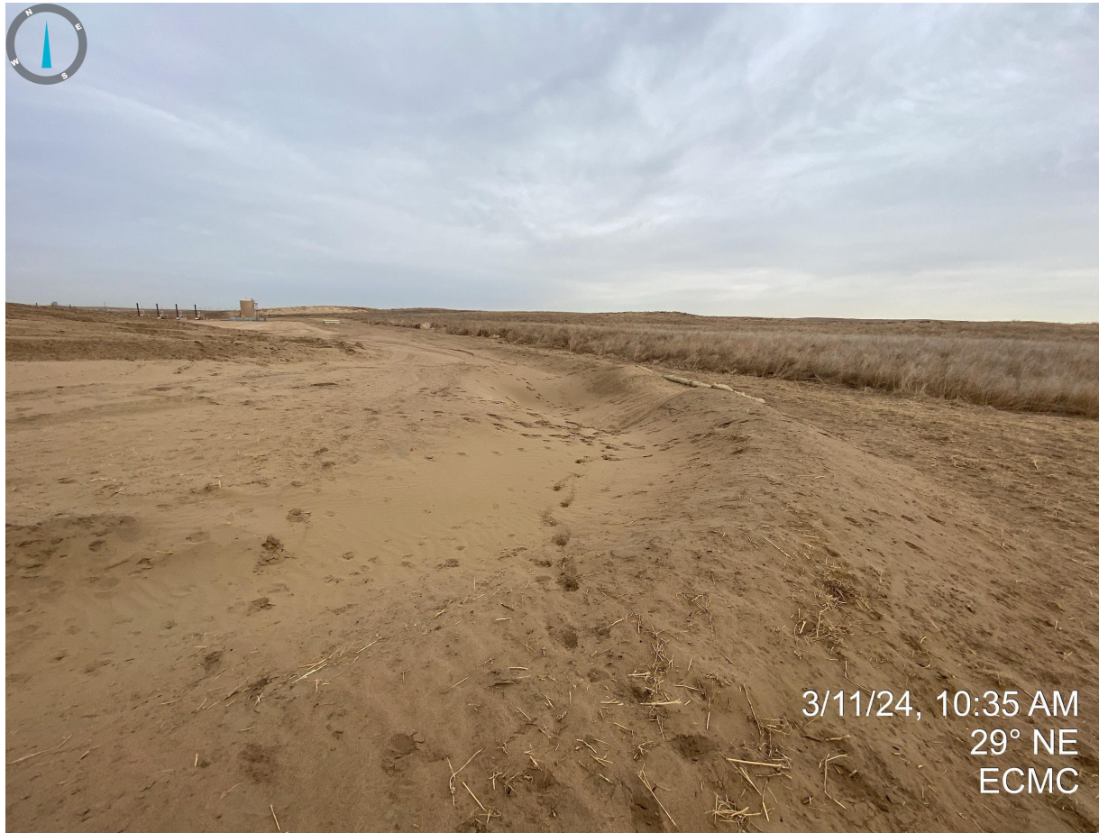
Photo 3. Southeast corner of location. A sediment trap has been installed on the perimeter of the location. Soils appear to be unstabilized with evidence of wind erosion and blown sand deposition. Additional stabilization BMPs are required on the loose soils.
