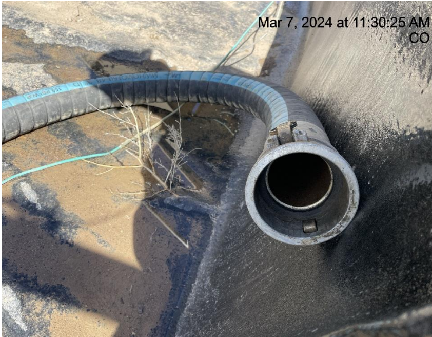
Photo # 9046 Open ended load line
