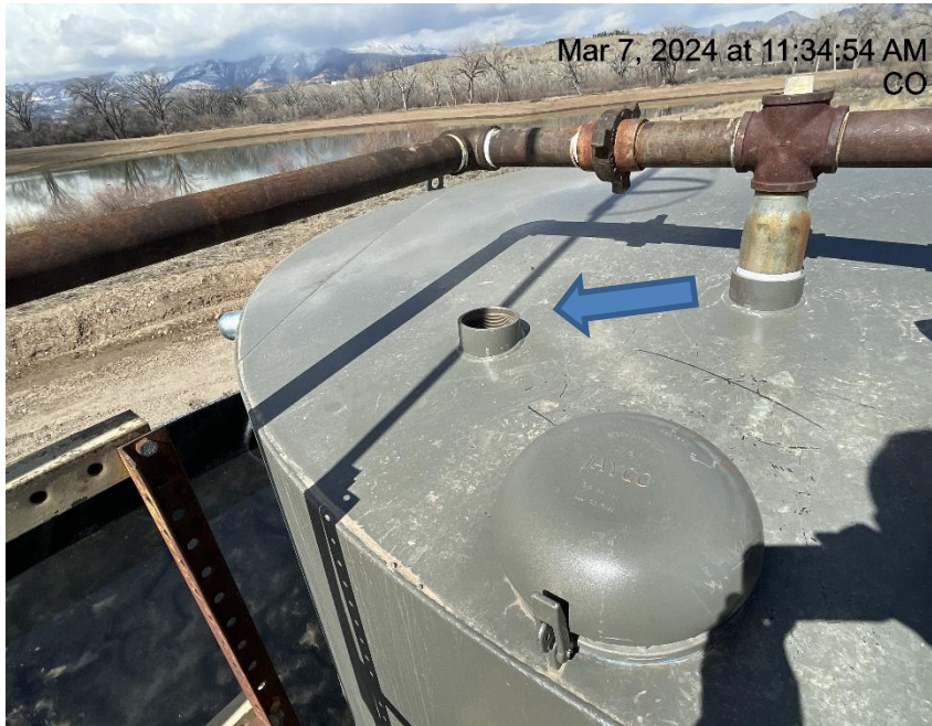
Photo # 9048 Open port on production tank/wildlife hazard
