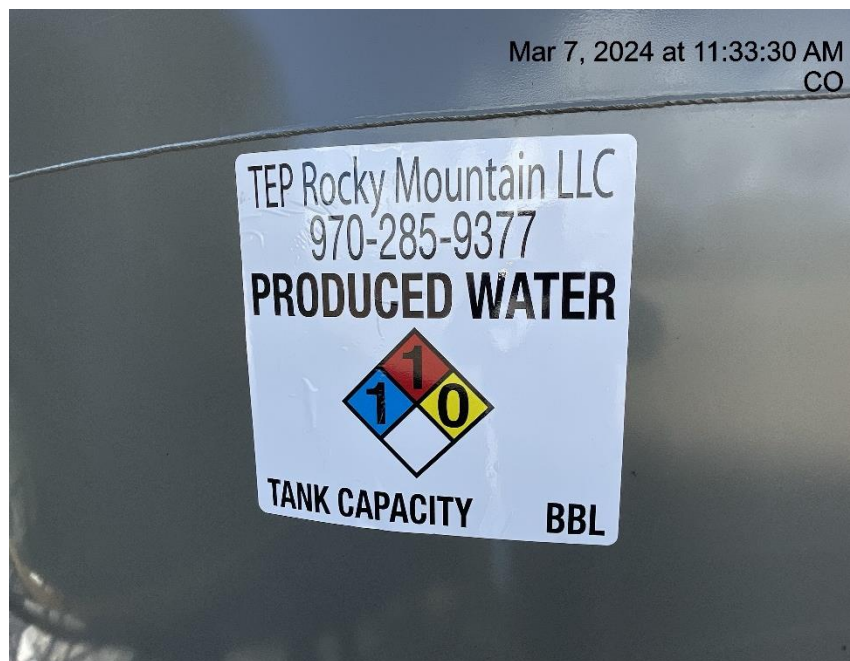
Photo # 9054 Tank label lacks required information
