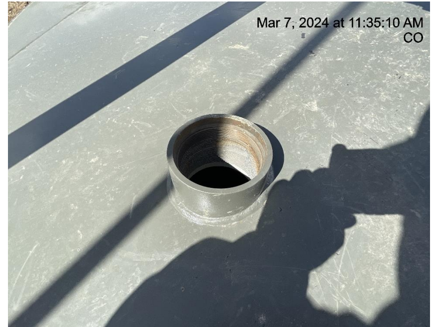
Photo # 9049 Open port on production tank/wildlife hazard
