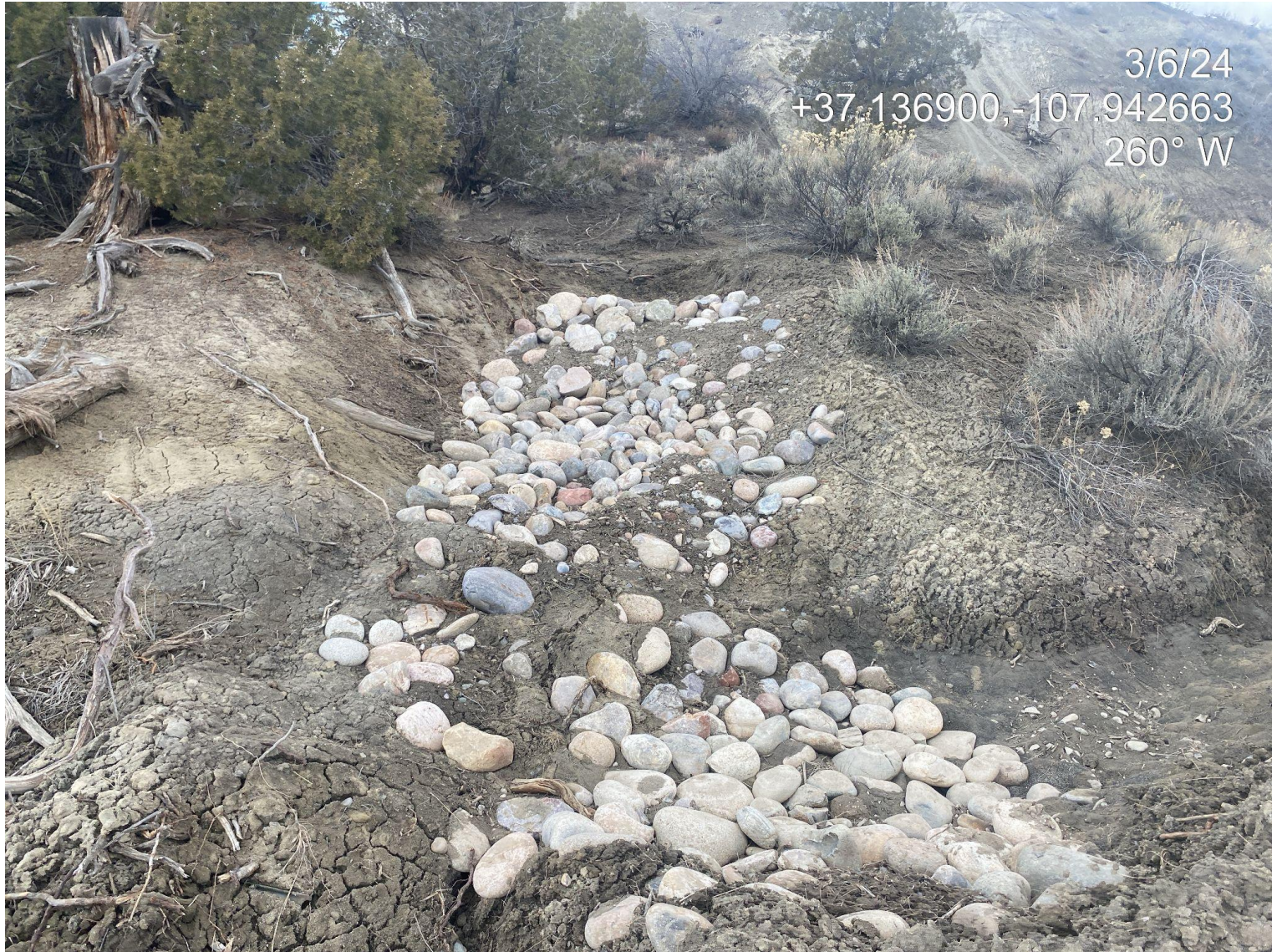
Photo 2. View of stormwater BMPs that are inadequate and have not been installed per good engineering practices.
