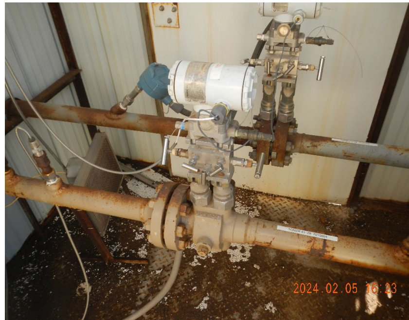
6. Gas meter inside meter shed.
