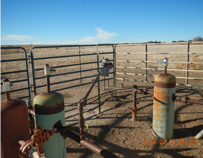
7. Domestic Tap connected to the inlet side of gas meter run flowline.
