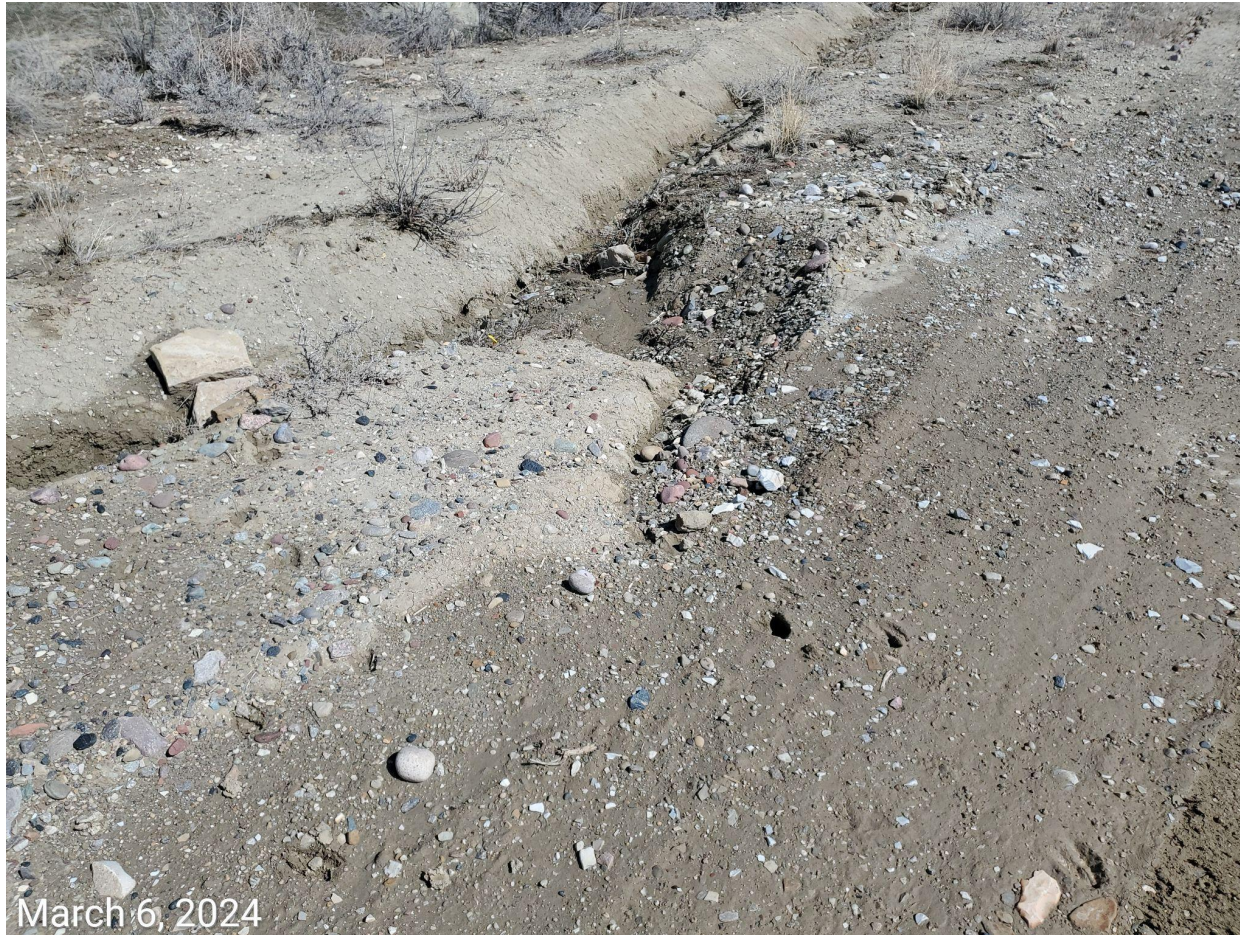
Photo 5: Erosion degradation has persisted along the access road and ditch.
