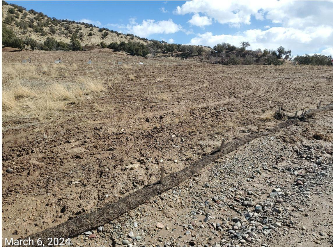
**Photo 4:** Photo taken from the western interim areas. Operator appears to have conducted additional work in these areas, however, stormwater and erosion control BMPs remain missing or insufficient. Erosion logs remain in disrepair. Photo also examples showing erosion logs on Location appear to have been constructed with a plastic material.
