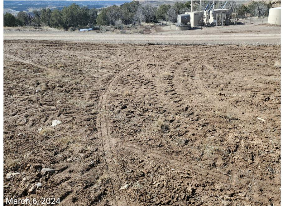
**Photo 3:** Photo taken from the western interim areas. Operator appears to have conducted additional work in these areas, however, stormwater and erosion control BMPs remain missing or insufficient; CA regarding interim reclamation remains outstanding.
