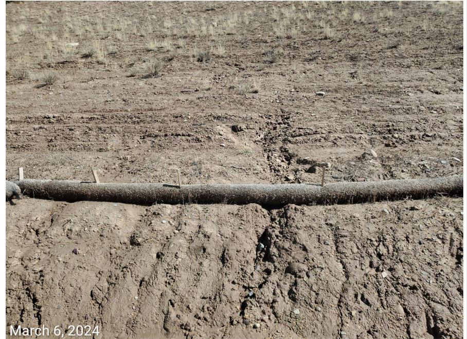
**Photo 1:** Photos taken from the eastern interim areas. Stormwater and erosion control BMPs remain missing or insufficient; erosion logs remain inadequate and not in proper functioning condition. Erosion degradation persists. CA regarding interim reclamation remains outstanding.
