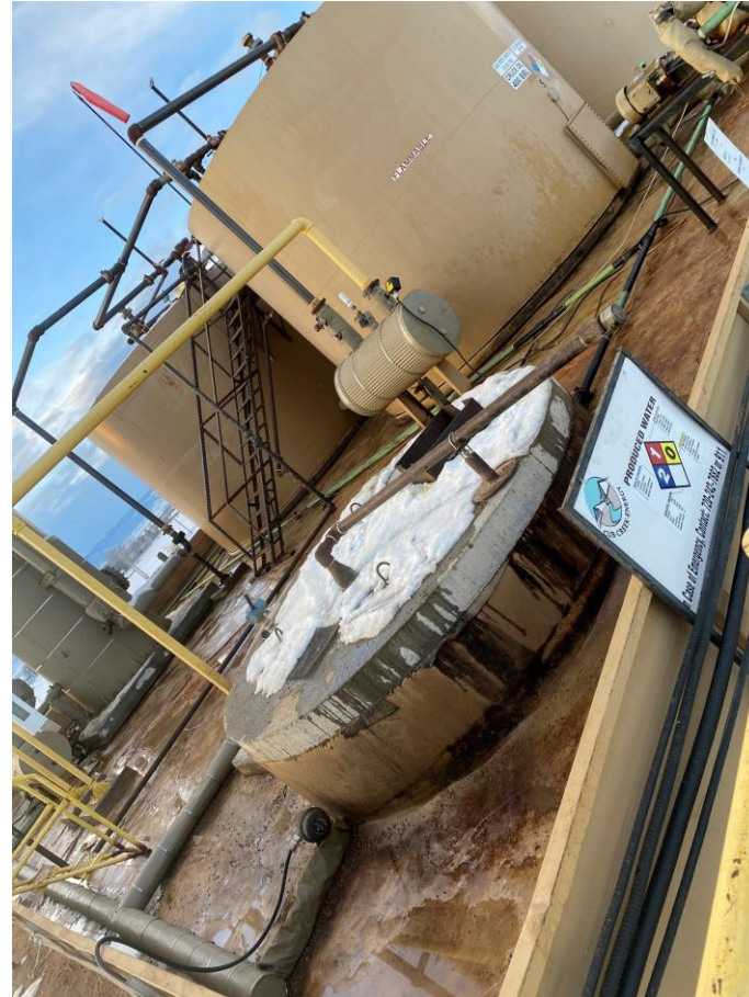
Inside of containment after hydrovac cleaning.
