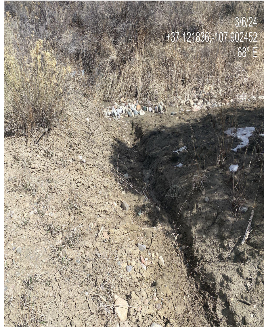
Photo 4. View of rill erosion forming in the southeast and northeast portions of the disturbance.
