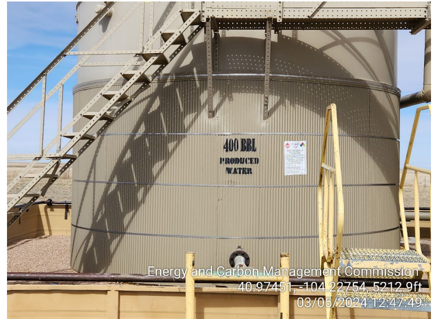
Photo 6 – NFPA Label missing on Produced Water Tank
