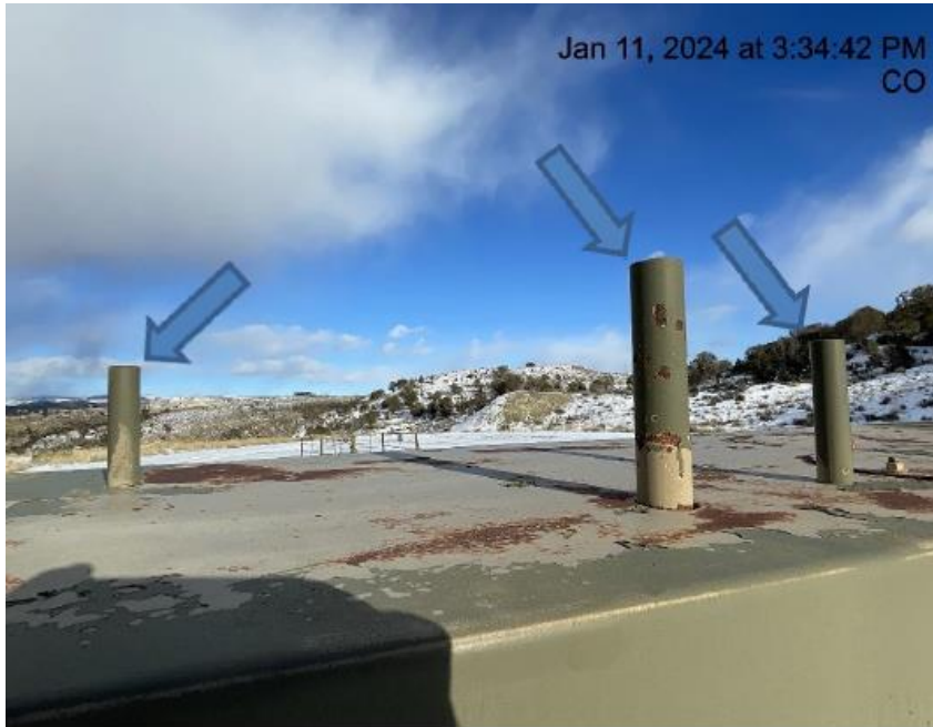
Photo # 2674 From inspection 708902787 conducted on 01/11/2024 PRV & rupture disc vent lines lack caps
