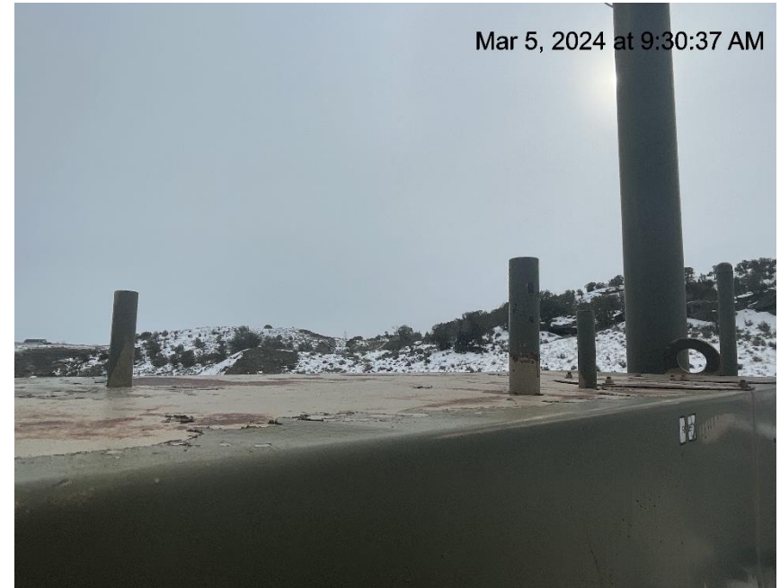
Photo # 8199 PRV & rupture disc vent lines lack caps
