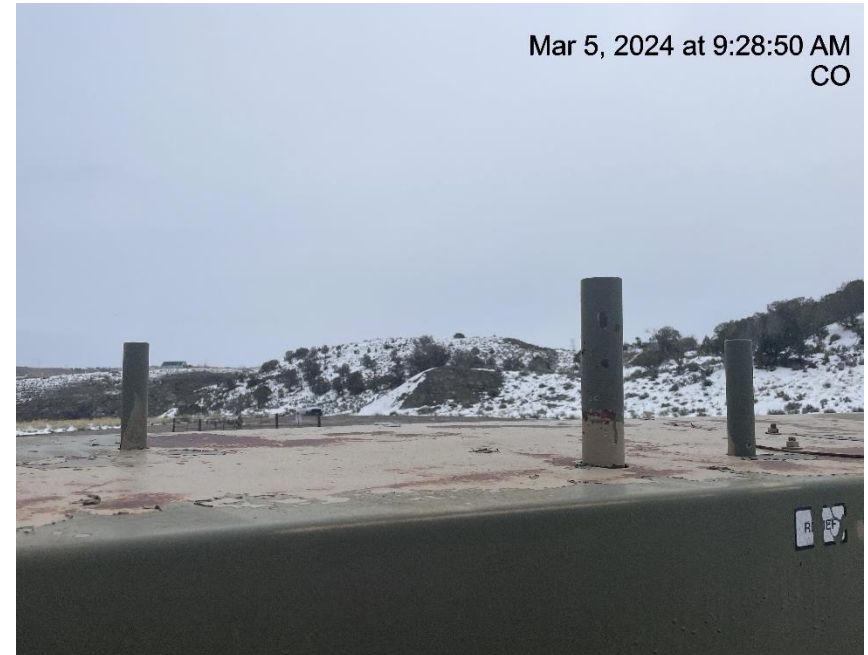
Photo # 8200 PRV & rupture disc vent lines lack caps
